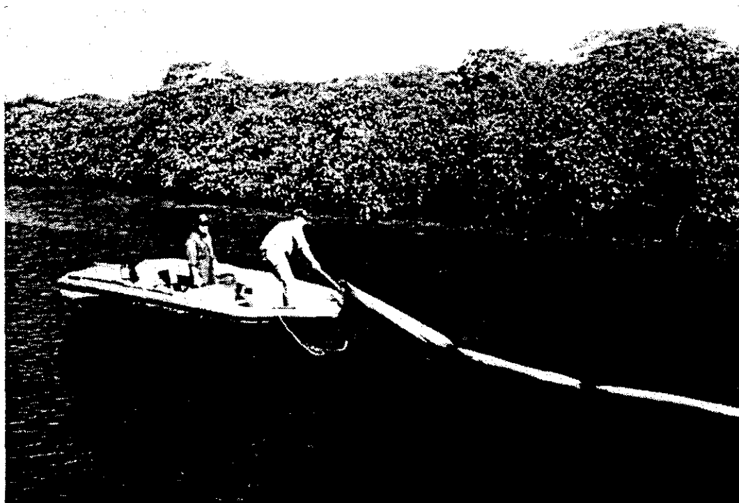
FIGURE 6. The booms extended out around the outer perimeter of the subtidal areas, creating an entirely enclosed area around the site.
