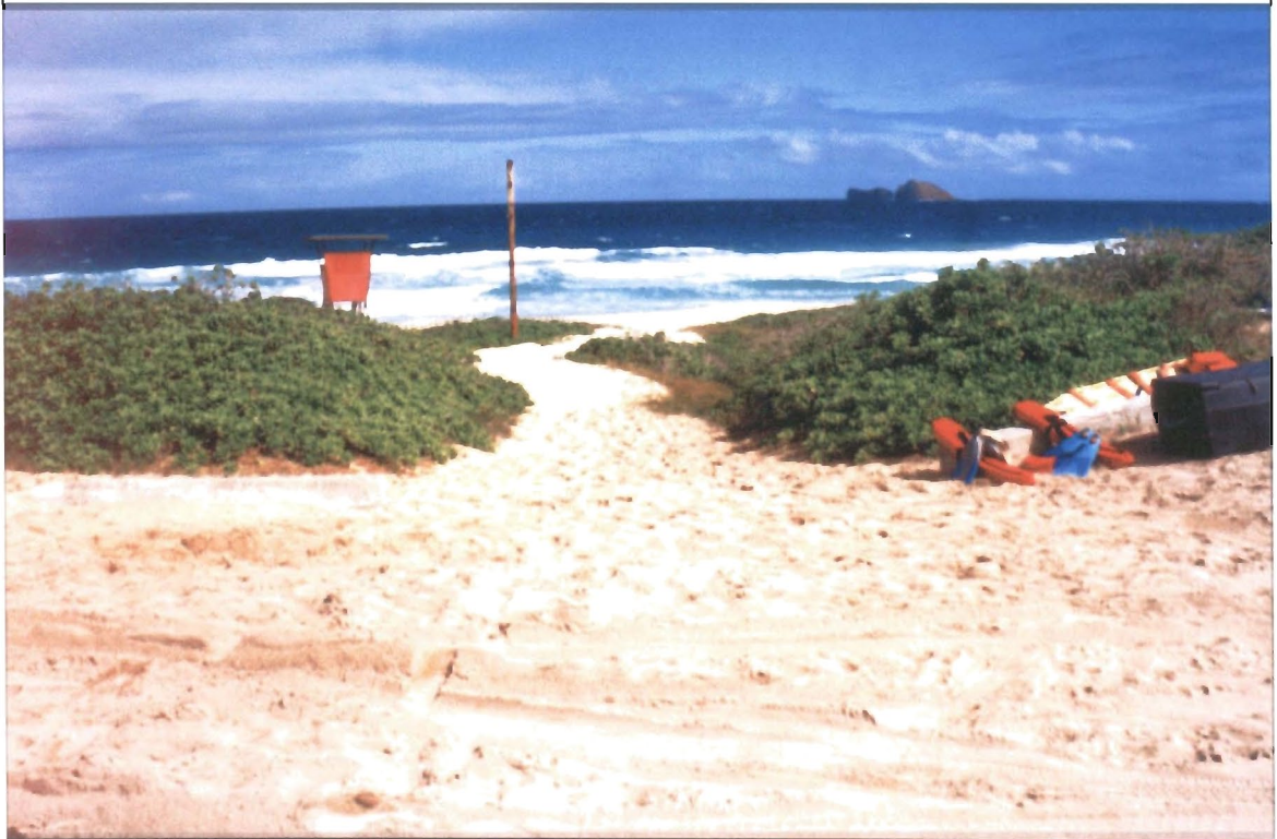
Photo 13. View of parking lot and path to beach through Naupaka at the Pyramid Rock Recreational Subarea. Note barely visible concrete barrier on the left that defines the seaward edge of the parking lot. Note also the quantity and depth of sand blown onto the parking lot. Vehicles are frequently stuck in this sand.
