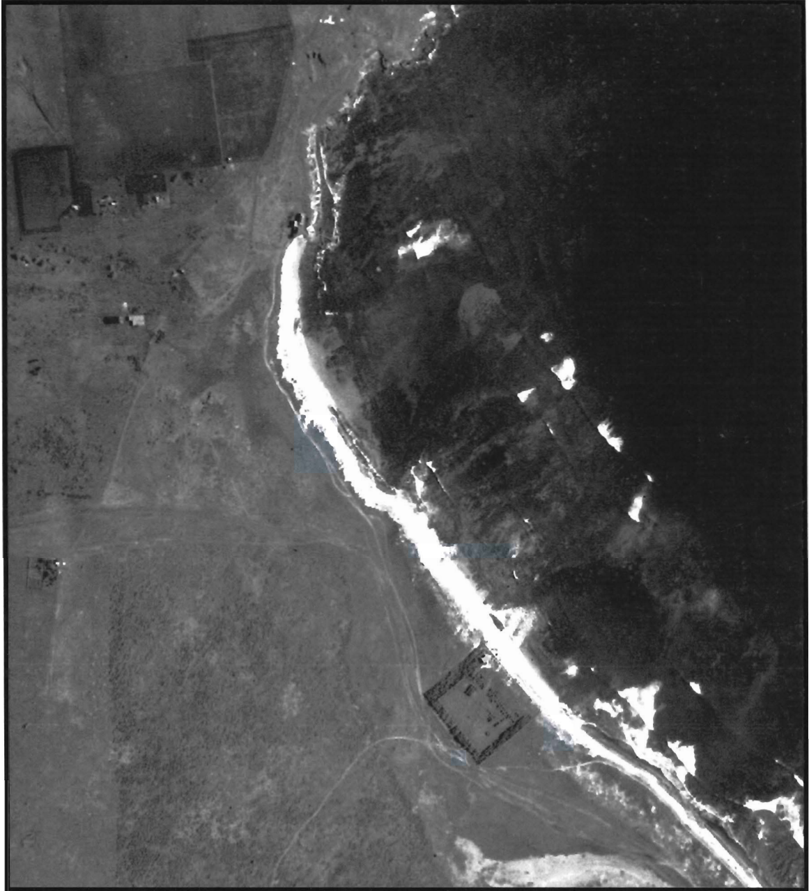
Figure 9. Fort Hase Beach Recreational Area. Aerial photograph taken by the U.S. Geological Survey in 1927. Note the lack of development in the coastal dune area with the exception of a road or track that parallels the shoreline in the approximate same location as the existing road.
