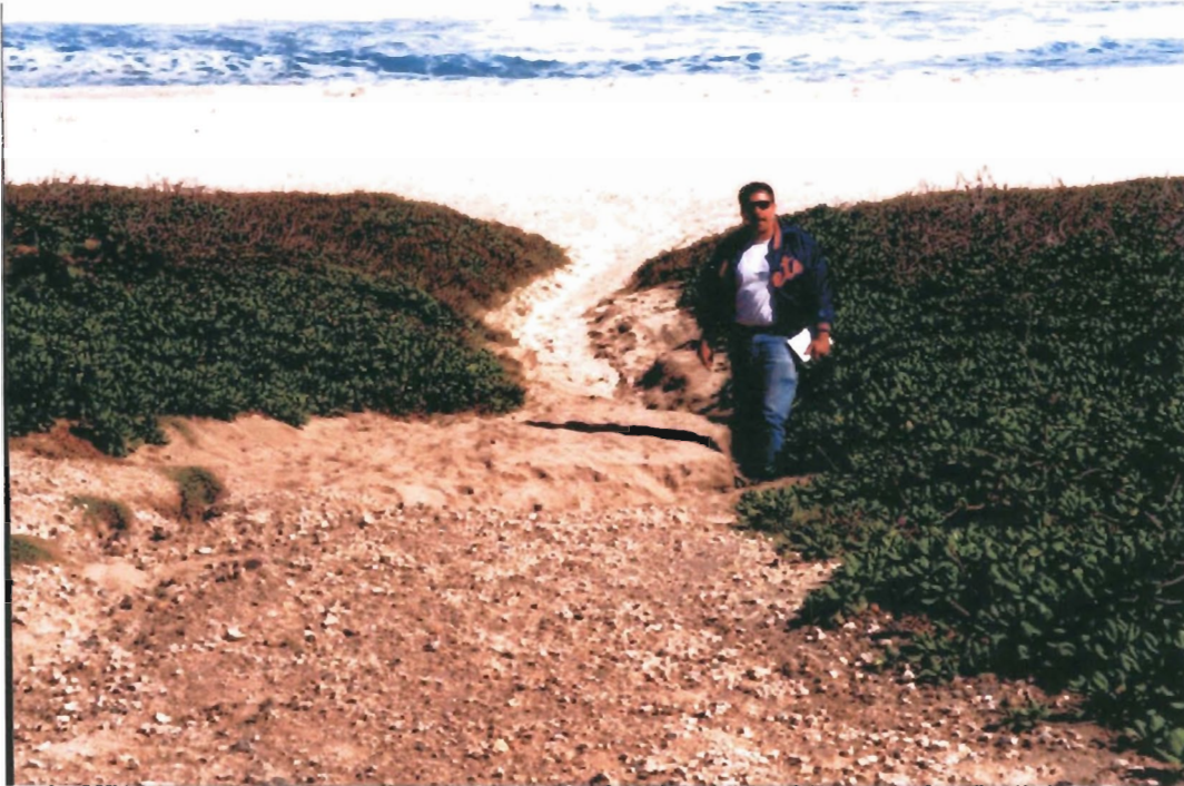
Photo 16. Erosion of pathway to the beach from the parking lot at Pyramid Rock Recreational Subarea. Note depth of gully.
