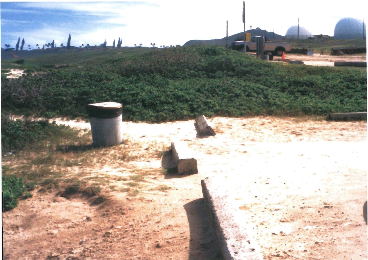
Photo 12. Concrete barricades to minimize (prevent) vehicle access to the beach at Pyramid Rock Recreational Subarea. Note movement of barrier toward beach and presence of sand blown into the parking area from the beach path.
