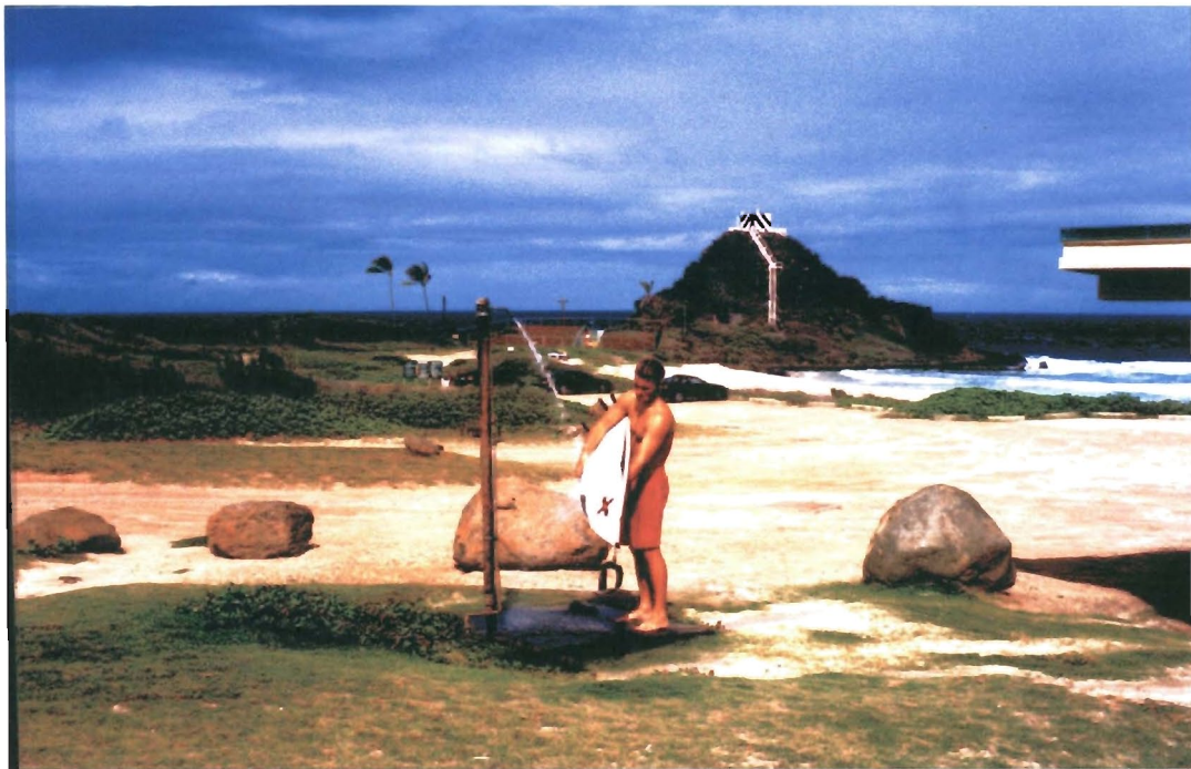
Photo 15. The shower at Pyramid Rock Recreational Subarea. Note the lack of a designated drainage channel. Water flows from the concrete shower pad across the coral limestone parking lot causing the development of eroded drainage swales across the parking area and through the upper beach dunes.
