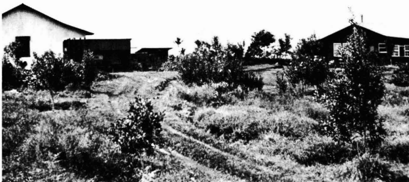
Figure 94. The Keauhou warehouse in Kona, built in the early 1930s, was already in bad condition when the authors saw it in the early 1950s.
