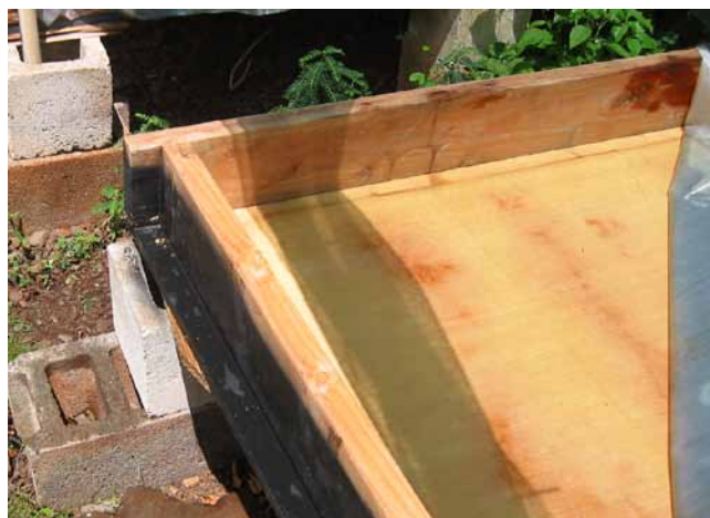
1. Lettuce tray corner, without plastic liner (2x6 side walls shown; 2x4s recommended)
