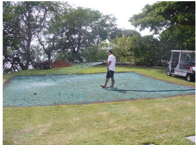
4. Application of hydromulch following stolonizing
