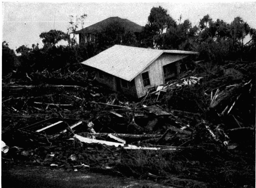
PLATE 3B. House in Keaukaha, east of Hilo, carried inland about 100 feet by the waves. The house in the background was above the reach of the water. Photo by G. A. Macdonald.
