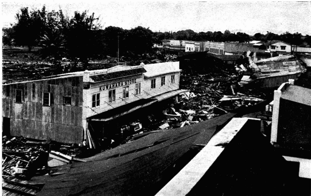
PLATE 3A. Wreckage left by the tsunami along Kamehameha Avenue, Hilo. Buildings on the left-hand (seaward) side of the street have been pushed into the street, some more or less intact, others as heaps of debris. Photo by Francis Lyman.
