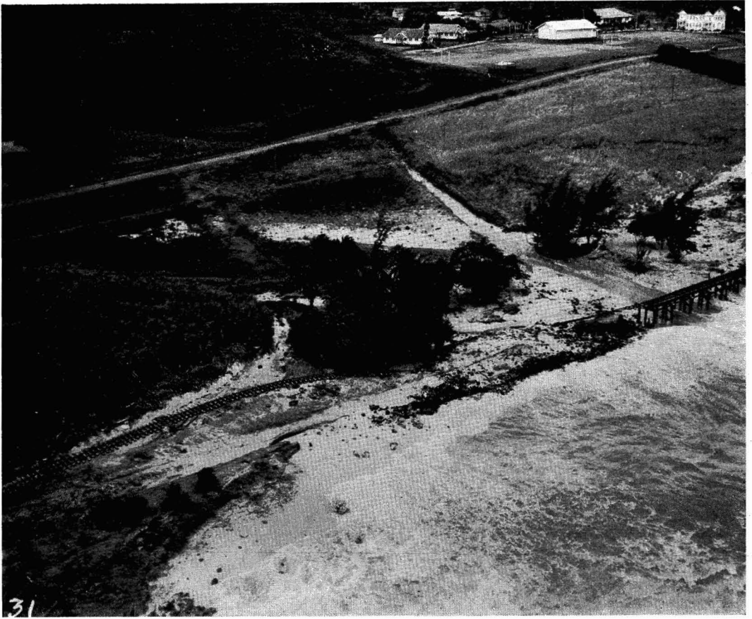
PLATE 6A. Railroad track swept inland from its bed at Waialeale, Oahu. Photo by U. S. Navy.
