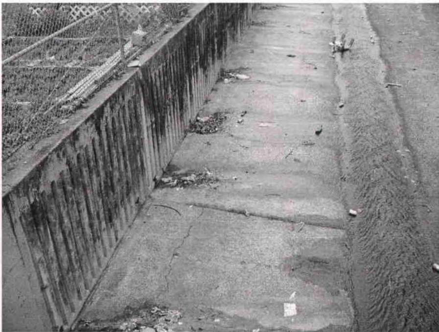
Appendix M. Pukele Stream channelization with trash debris fanning out from small drains along channel floor. View from Ahe St. Bridge looking downstream
