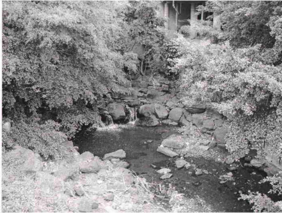
Appendix H. Palolo Stream semi-natural channel. View from St. Louis Dr. Bridge looking upstream
