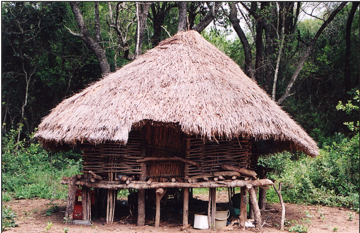
Figure 6. A maize store built like a miniature house with a thatched roof in the community of Manqakulane, Maputaland, KwaZulu-Natal province, South Africa, as established by a survey in 2002.
