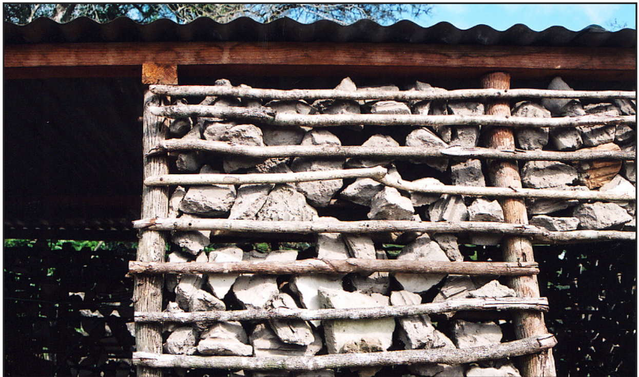
Figure 5. An example of a wood and stone wall, with the space between the horizontal wooden laths filled with old concrete rubble. Community of Manqakulane, Maputaland, KwaZulu-Natal province, South Africa, as established by a survey in 2002.
