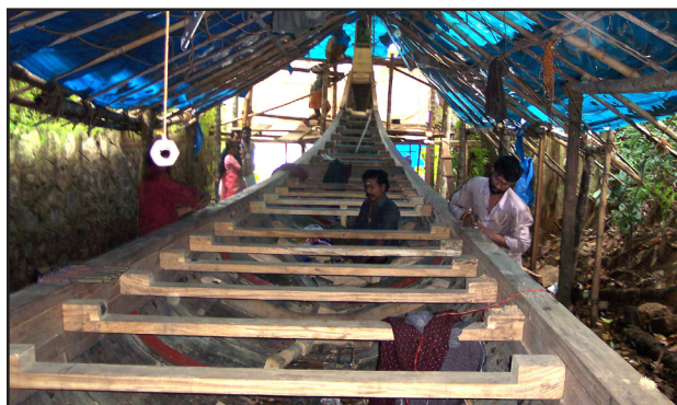
Figure 28. A new construction of a snake boat.
