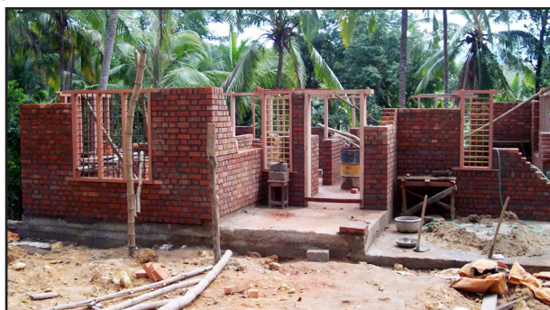
Figure 16. A modern construction with doors and window frames made of wild jack wood.
