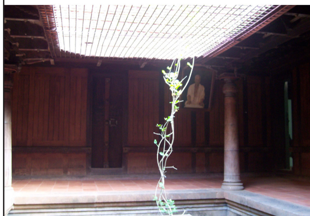
Figure 15. A traditional building ( nalukettu ) made of wild jack wood with wooden pillars and walls.
