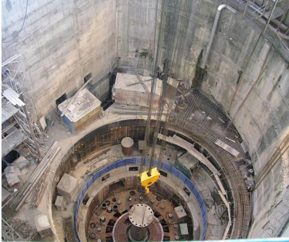
Fig. 6. The hydraulic unit shaft
