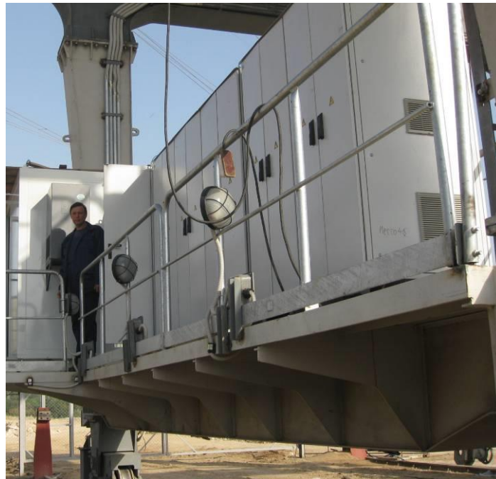
Fig. 9. Crane control device placement
