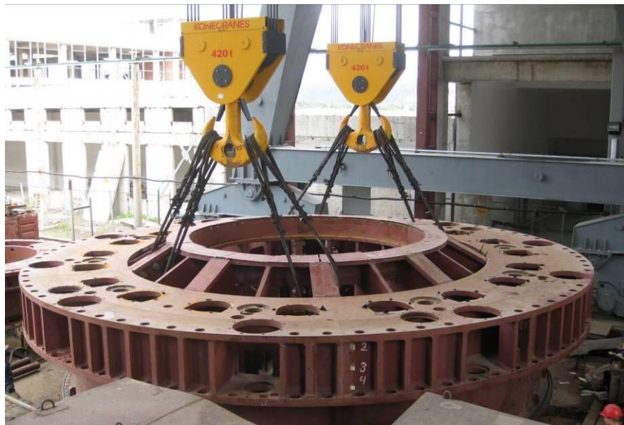
Fig. 8. Framework of the hydraulic units
