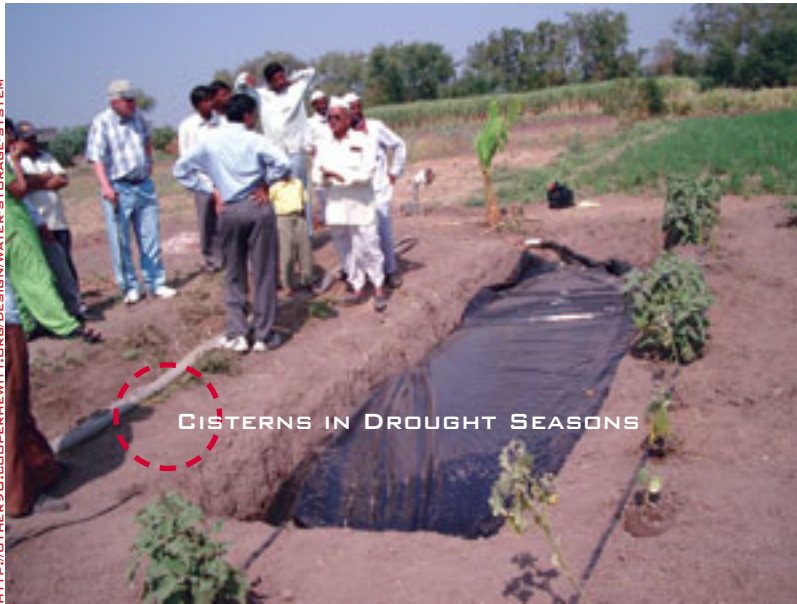
○ Plastic bag cistern developed for countries within India, Africa, and the Middle East.
