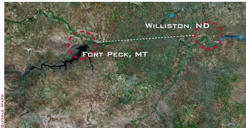
○ An aerial perspective of Fort Peck Dam in Montana with its proximity to Williston, North Dakota.
