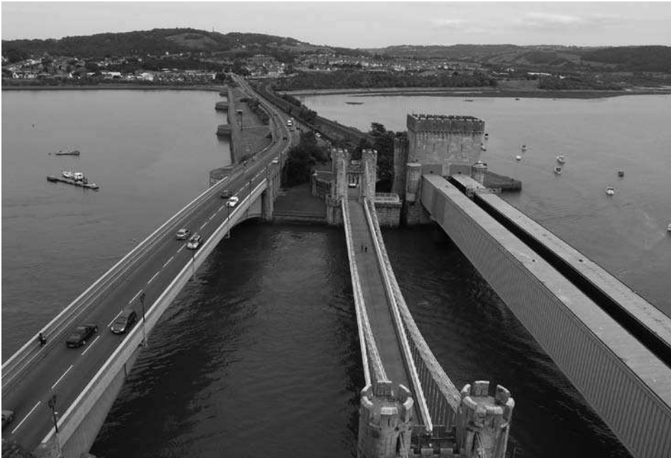
Conwy Bridge, North Wales.
