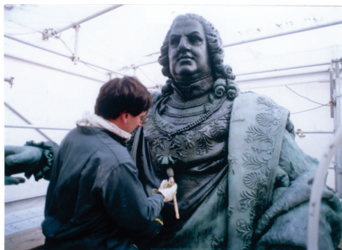
Figure 5. Coating of a bronze statue by applying microcrystalline wax on the cleaned surface.
