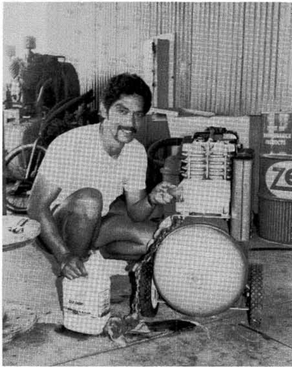
Henry Hua adds oil to an NELH air compressor during maintenance service.
