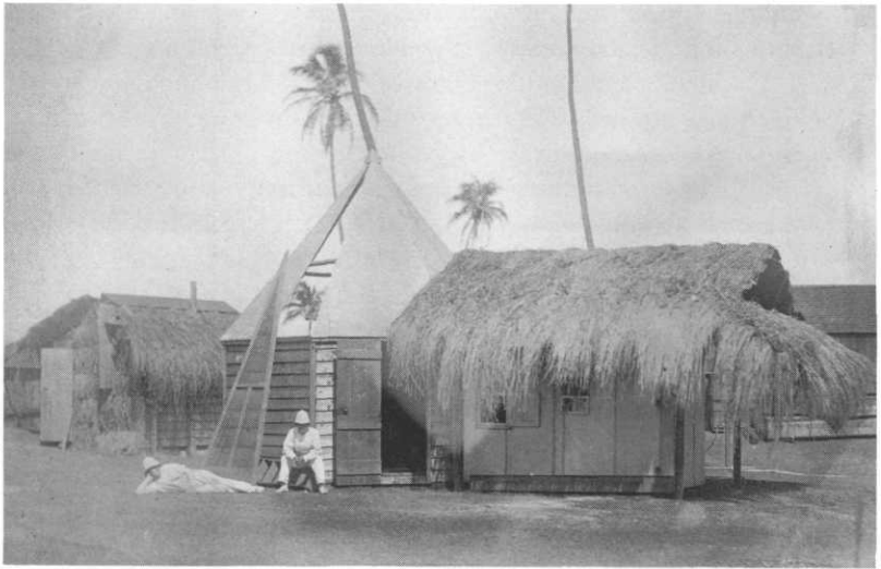
FIG. 5. Transit hut and photo hut, Honolulu, with roofs partially covered with rushes to counter the tropical heat. (RGO archives, Cambridge University Library.)
