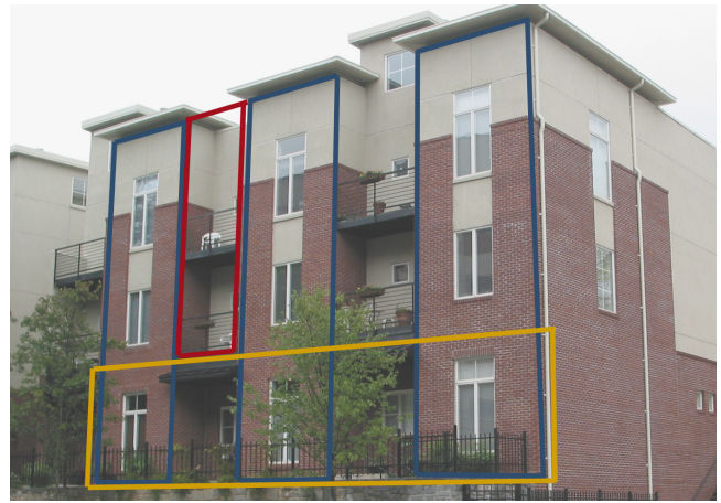
Figure 3: Photograph of a building which shows vertical coherence (balconies and material) and horizontal coherence (window styles).
