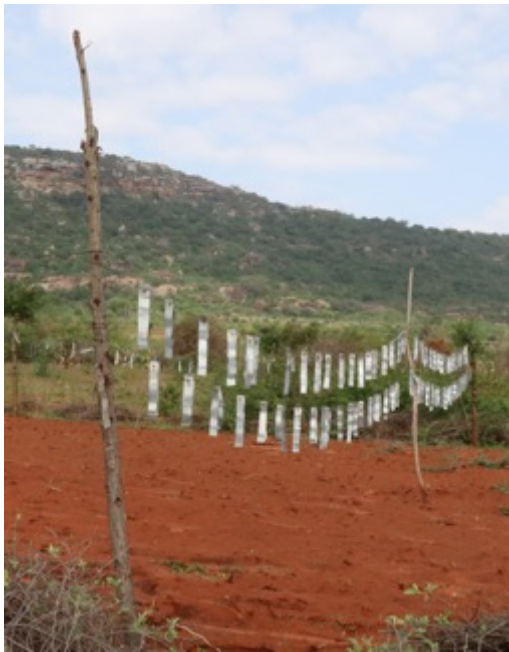
Figure 2. A double Kasaine metal strip fence, constructed and erected in the farming community of Sasenyi, Kenya. Photo taken by Sophia Corde.
