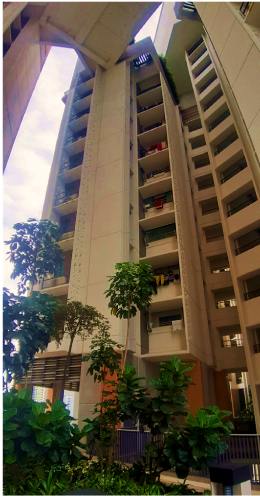
Fig. 6. Vertical Breezeway type (VB). Skyville@Dawson (SV) building.
