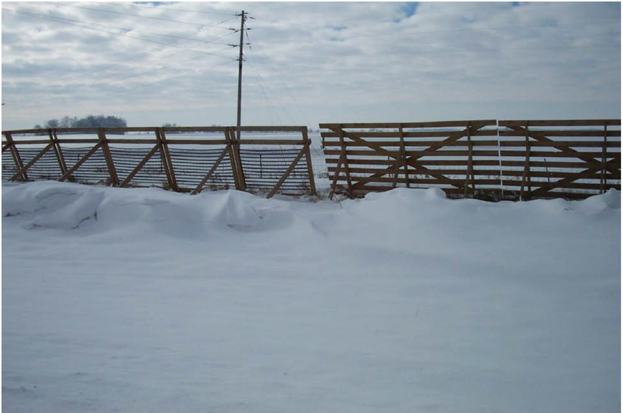
Figure 9.3 Structural Snow Fences at Wolcott Evaluation Site (Left Tensar – Right Wyoming)
