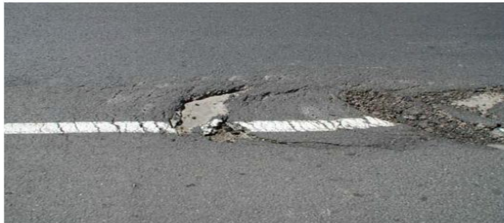
Figure 7: Slippage Cracking
