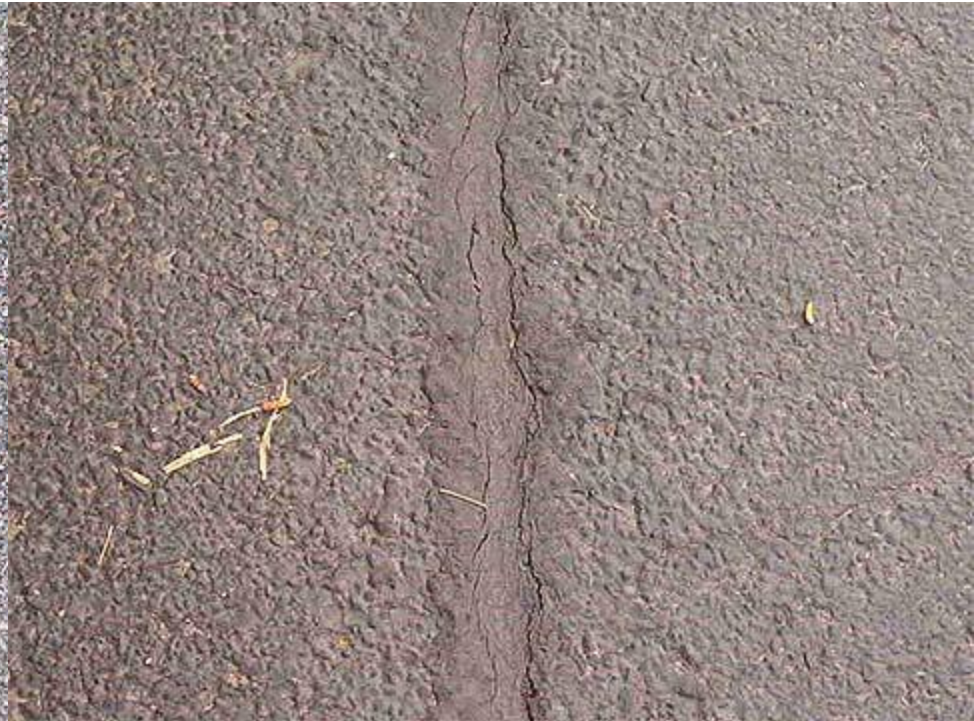
Adhesive Failure
