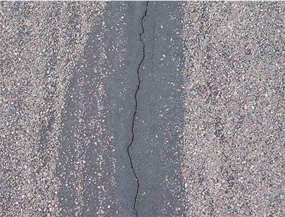
Cohesive Failure
