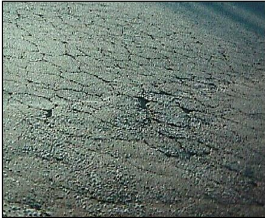
Figure 1: Fatigue Cracking
