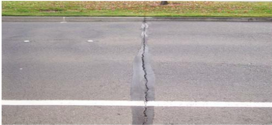
Figure 5: Reflection Cracking
