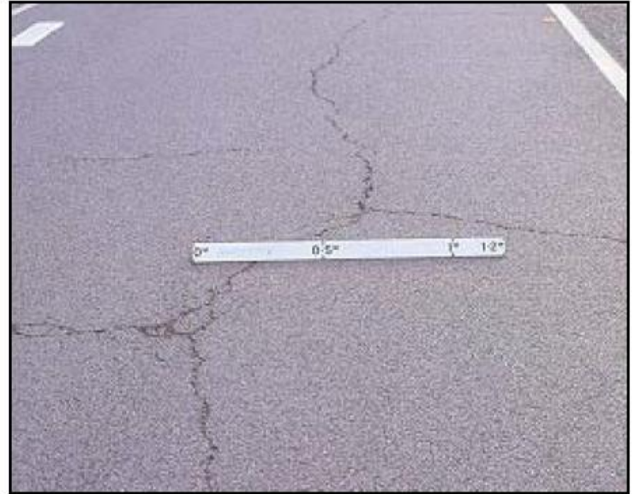
Figure 4: Block Cracking
