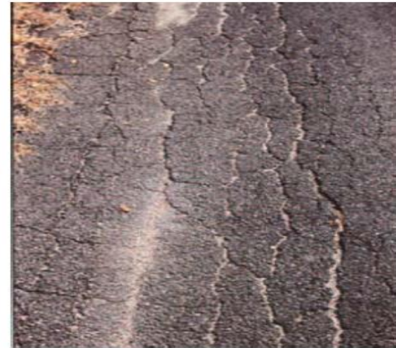
Figure 6: Edge Cracking
