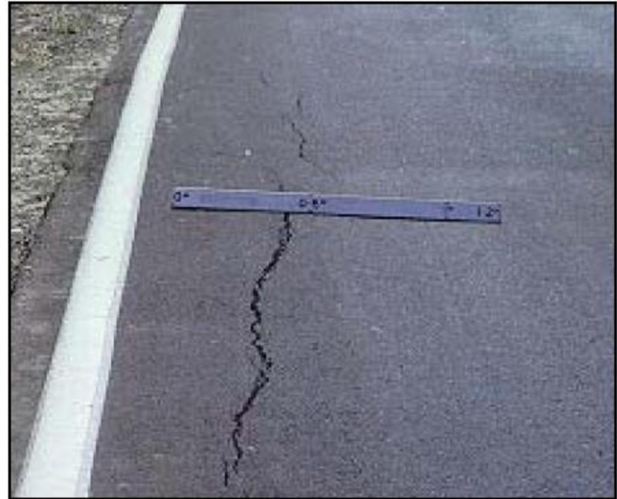
Figure 2: Longitudinal Cracking
