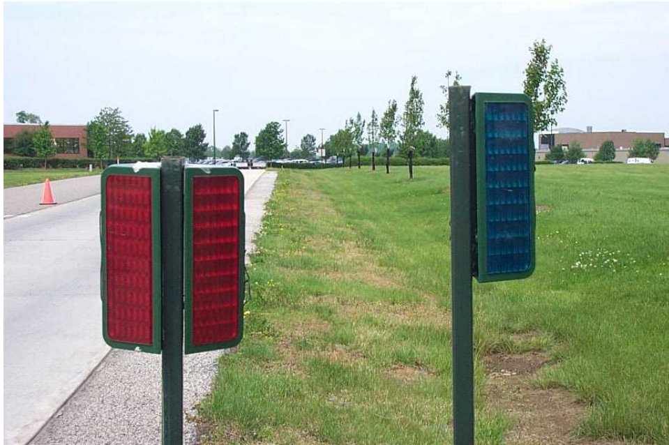
Figure 5. Single and Double Reflectors
