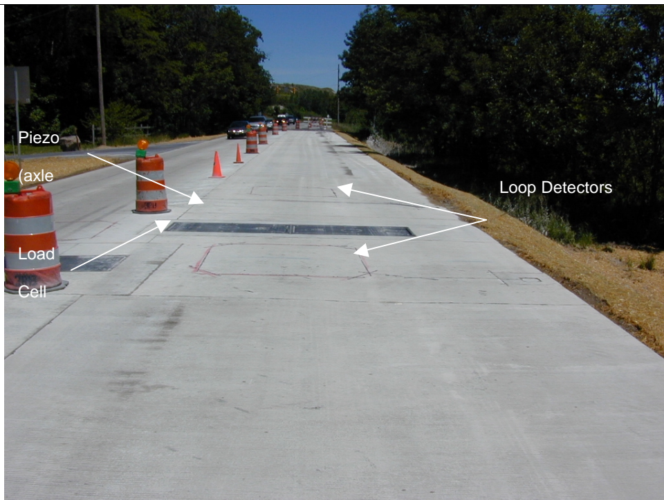
Figure 2: WIM scales (during construction ~July 2001).
