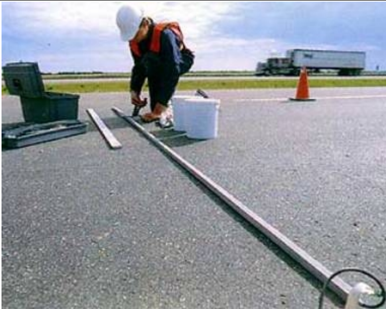
Figure 3-3: A technician installs a piezo-electric sensor
