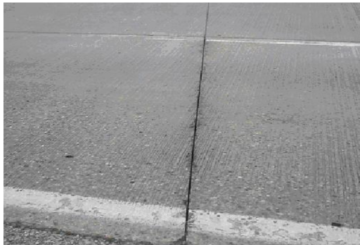
Figure 6-14 Joint Condition after Sealant Removal
