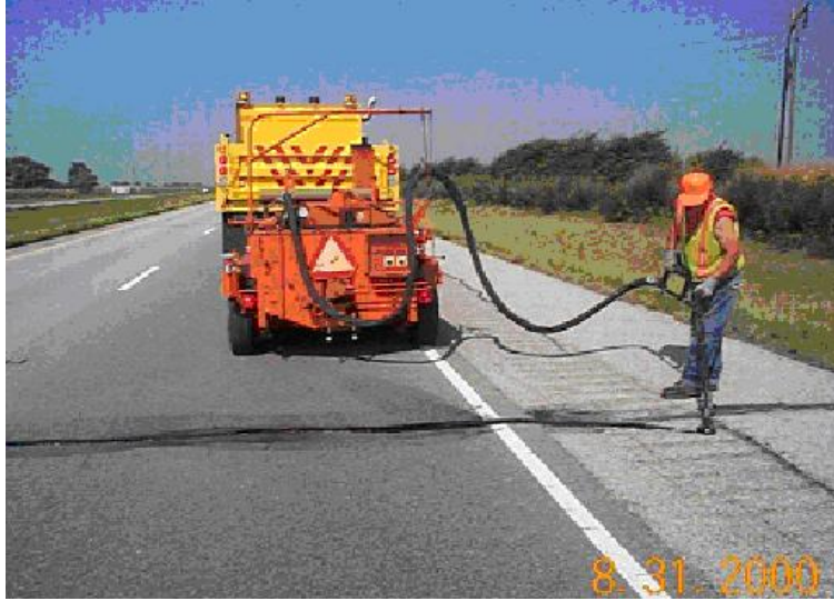
Figure 6-7 Crack Sealing Operation
