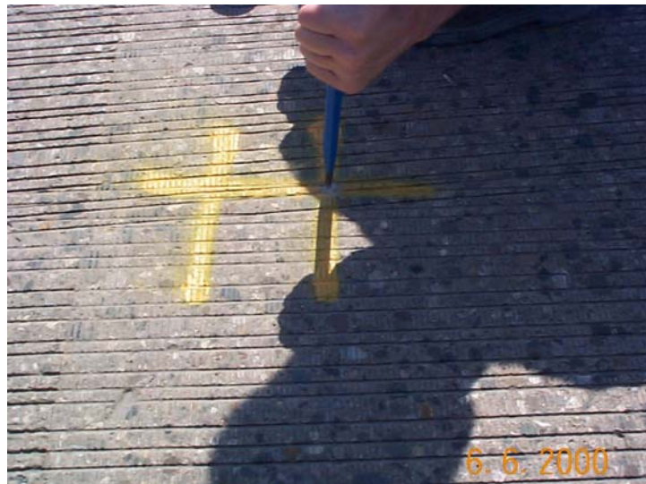
Figure 6-24 Marked Test Spot
