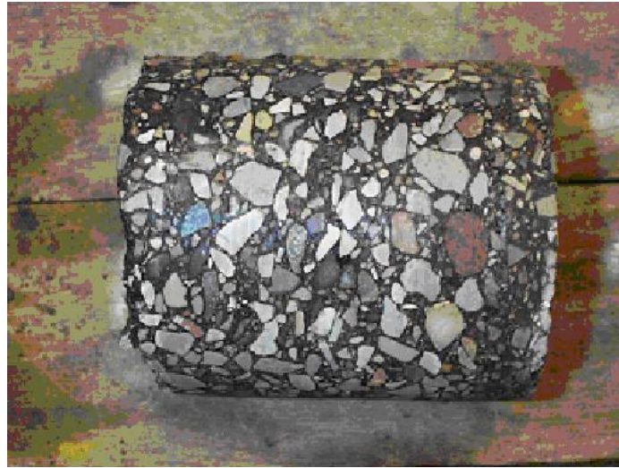
Figure E-1 Pavement Core on Northbound SR25
