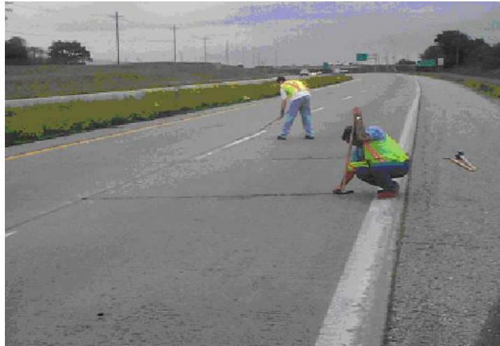
Figure 6-13 Sealant Removal Operation
