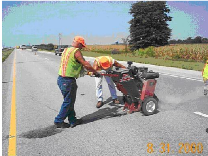
Figure 6-17 Crack Routing for Unsealed Section
