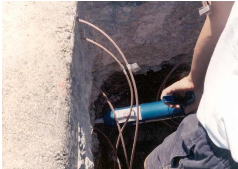
Figure 3.17 -- Sealing the sensor drill holes
