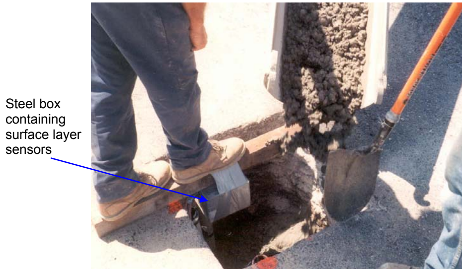
Figure 3.18 -- Backfilling the instrumentation pit with PCC
