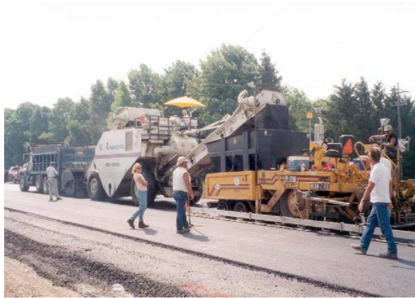
Figure 3.14 -- Pavement laydown operation
