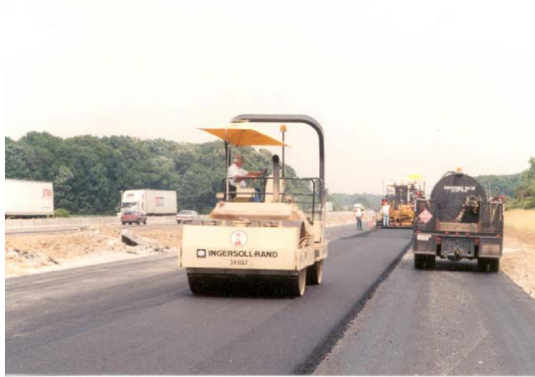
Figure 3.15 -- Pavement compaction operation
