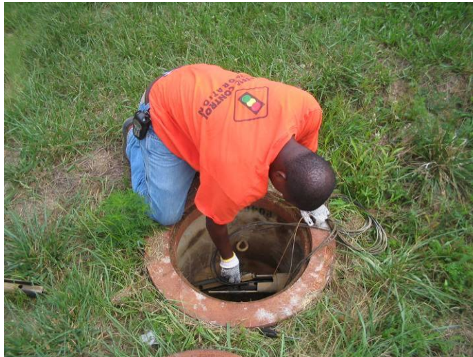
Figure 8.4 3M Microloop Sensors Placed at correct depth for ease of maintenance access
