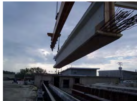
h) Removal of prestressed beam from form
