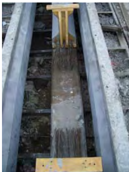
g) Strands after flame cutting
