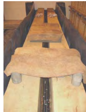
g) Curing pool (note the perforated garden hoses between the beams)
