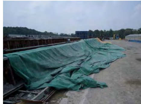
f) Curing of prestressed concrete specimens
