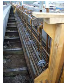
d) Final view of reinforcement before closing of forms
