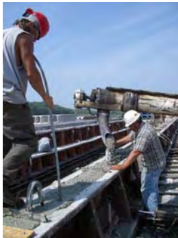
e) Casting and consolidation of concrete
