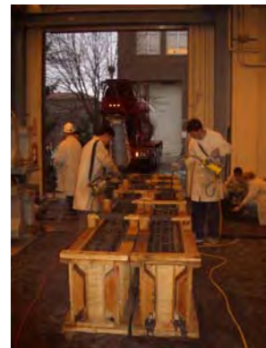
e) Consolidation of concrete
