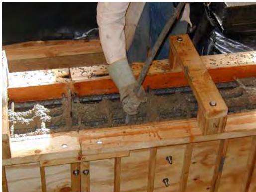
f) Cast and consolidation of beam for Specimen 13.3-2.6-98 and Specimen 13.3-5.4-98
