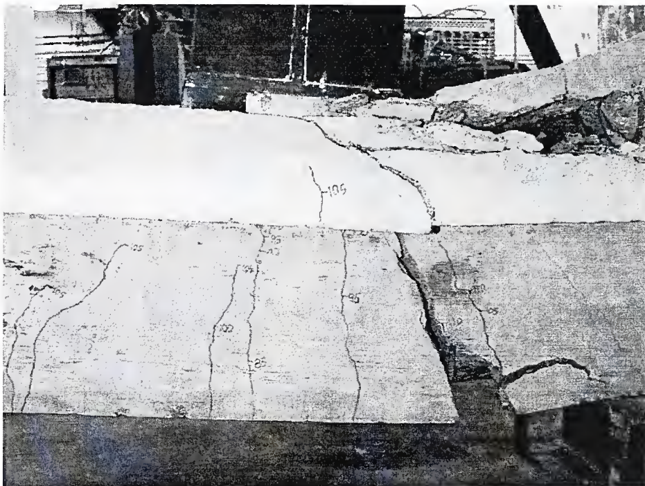
T-Beam FWC-6" Stirrup Spacing (North Face)
