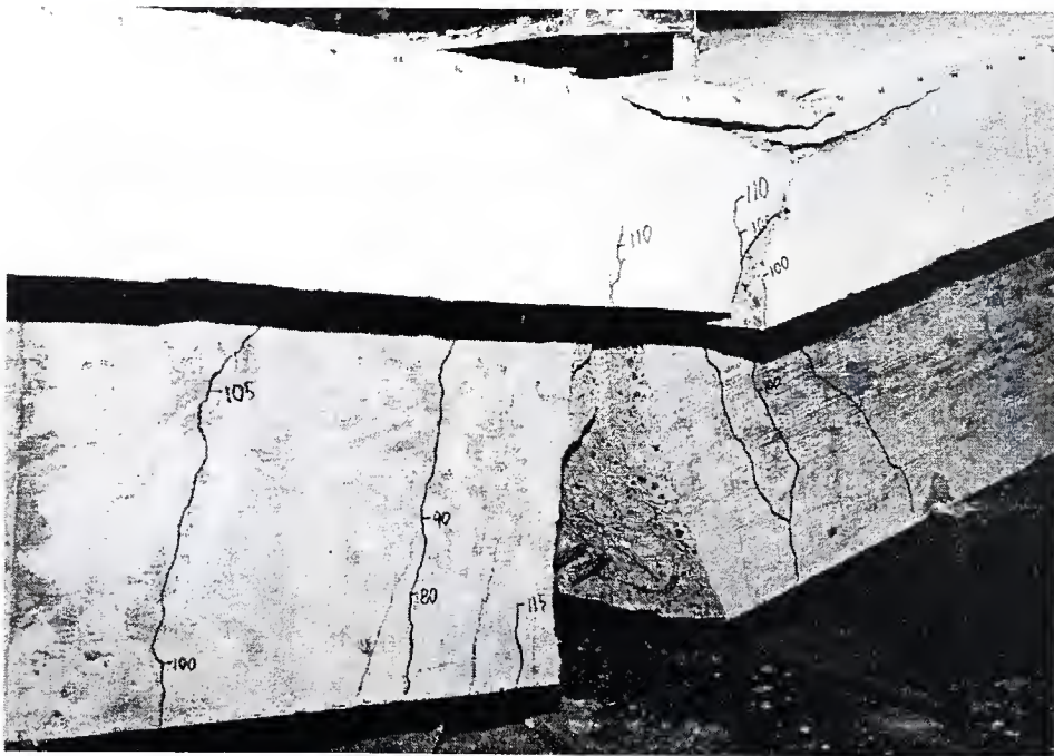
T-Beam FWC-3" Stirrup Spacing (North Face)
