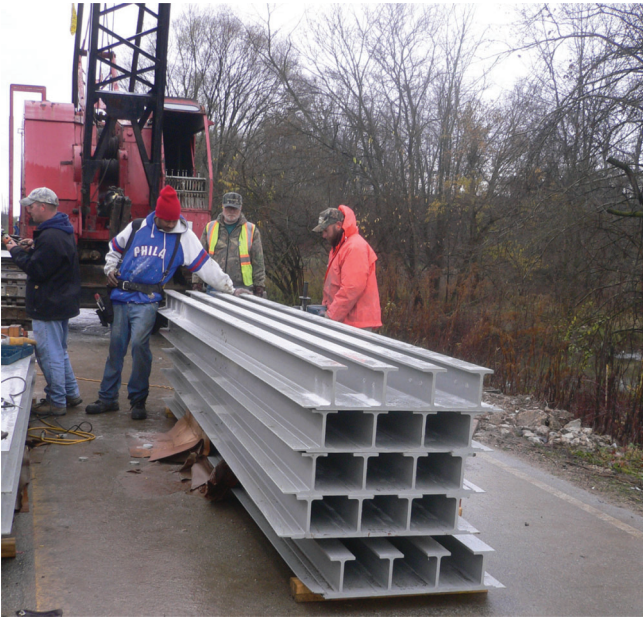
Figure 5.50: View of Bottom Deck Sections
