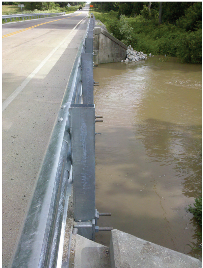
Figure 5.66: Guardrail and Sugar Creek
