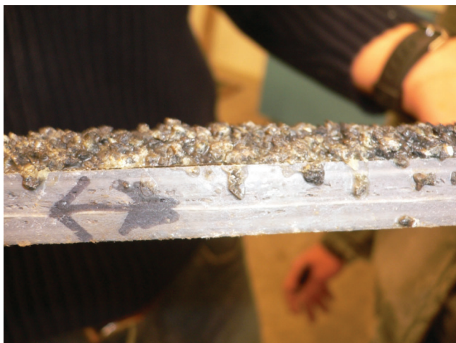
Figure 6.21: Delamination Between Wearing Surface and FRP Plate
