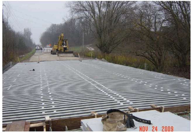
Figure 5.59: Foam Dams in Place at Girder Lines and Guardrail Connection Locations
