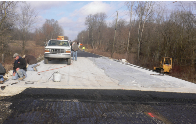
Figure 5.63: Protective Tarp on Deck Without Wearing Surface; Work on Approach Spans
