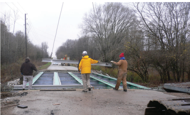
Figure 5.52: Placement of an FRP Deck Panel on Girders
