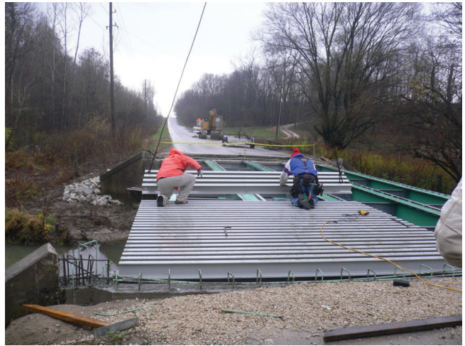
Figure 5.53: Placement of an FRP Deck Panel on Girders
