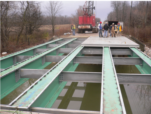
Figure 5.51: View of Girders Prepared with Angles for Grouted Haunches
