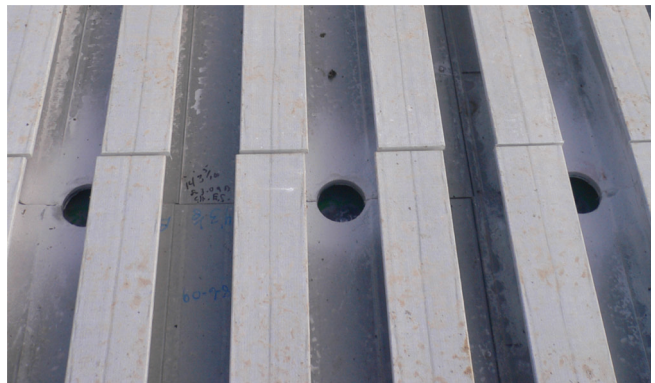
Figure 5.54: Bottom FRP Deck Sections at Crown Connection with Holes for Shear Studs
