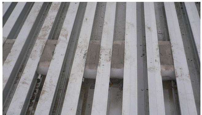
Figure 5.61: Grout Pockets After Grout Placed
