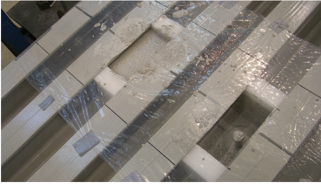
Figure 5.12: Deck to Girder Connectors (embedded in non-shrink epoxy grout)
