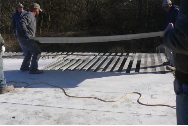
Figure 5.62: Placement of FRP Top Plate
