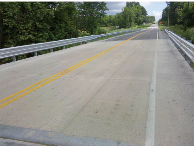
Figure 5.64: Finished Bridge with Wearing Surface and Guardrails
