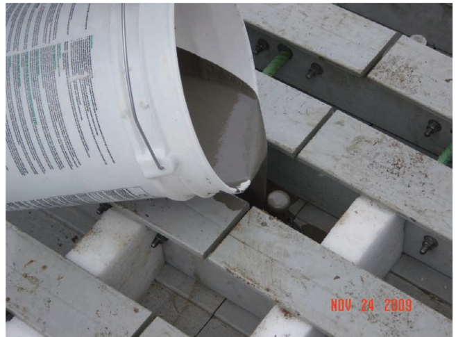
Figure 5.60: Placement of Grout in Shear Stud Grout Pocket
