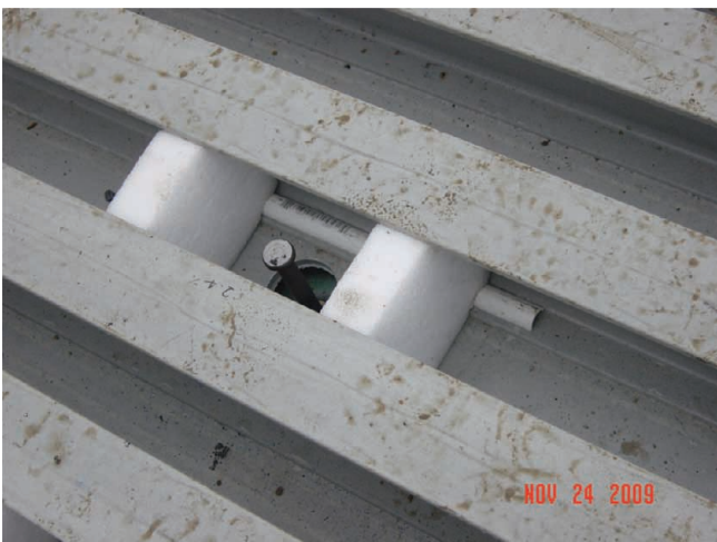
Figure 5.58: Tube to Allow Water to Flow Through Pocket After Grouted
