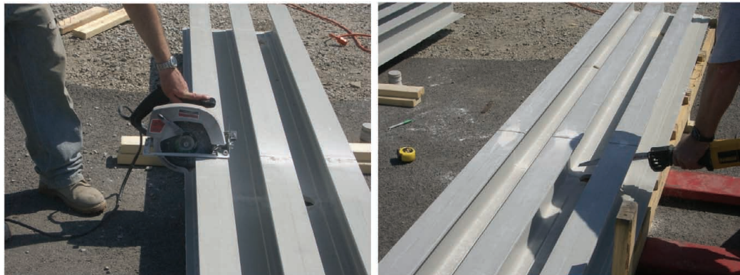
Figure 5.7: Cut at Center of Bottom Section
