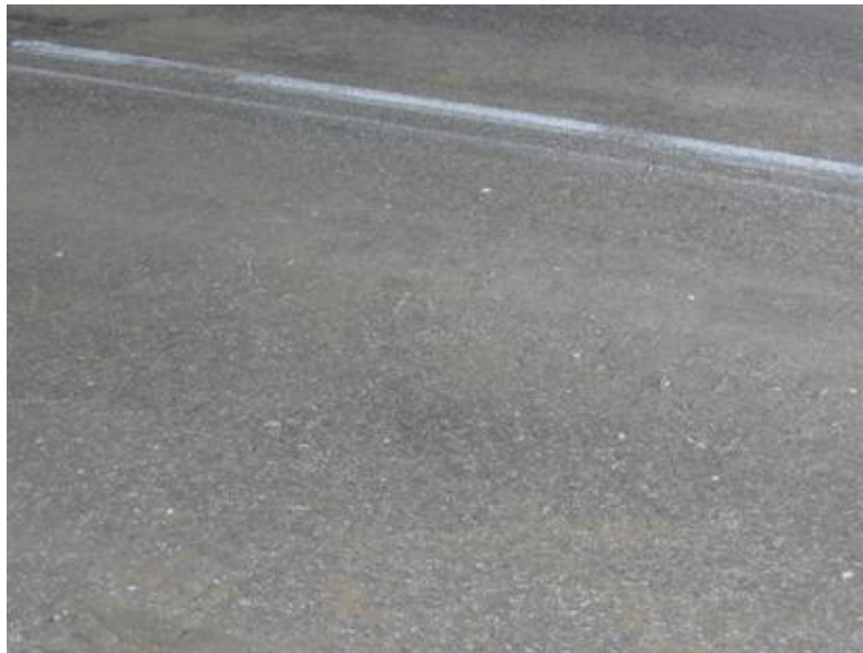
Figure 5-1 Surface of the Tested Asphalt Pavement
