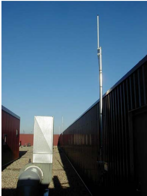
Figure D-2: (Top) View of MSEE building showing three testbed antennas over the roof-line. (Bottom) View of testbed antennas from on the MSEE roof.
