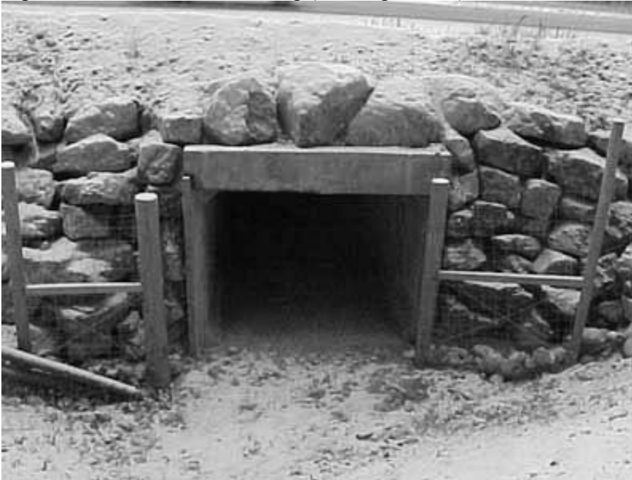
Figure 3. Box culvert and fencing (Clevenger 2004).
