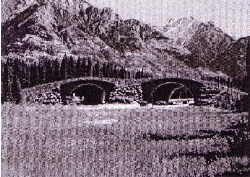
Figure 7. Overpass in Banff National Park, Canada (CPAWS 2004).
