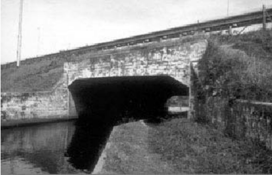
Figure 6. Box culvert modified with ledge for small animal passage (Bank et al. 2002).
