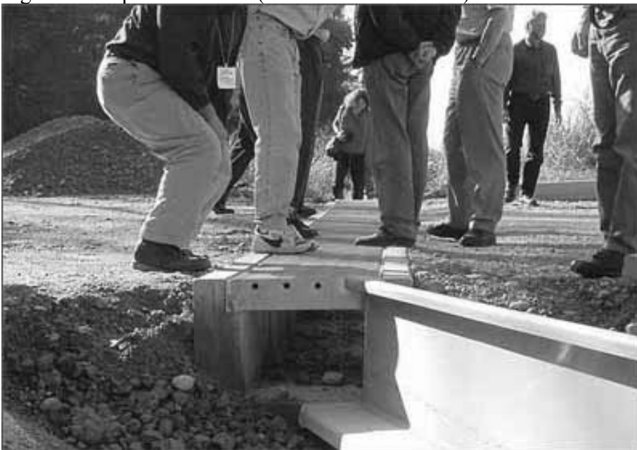
Figure 2. Amphibian tunnel (FWHA/USDOT 2002).
