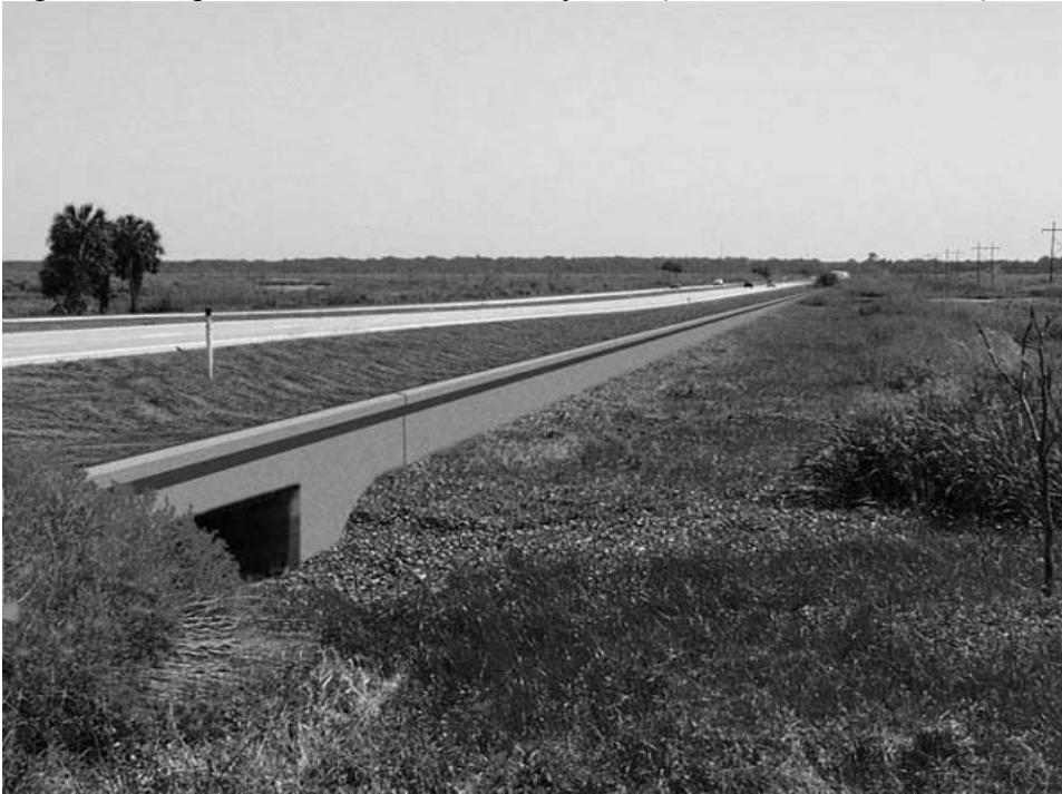
Figure 9. Amphibian wall and culvert system (FWHA/USDOT 2002).
