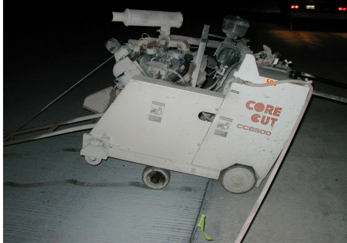
Figure 3.14: Conventional wet cut 65 horsepower saw with 20” diamond blade
