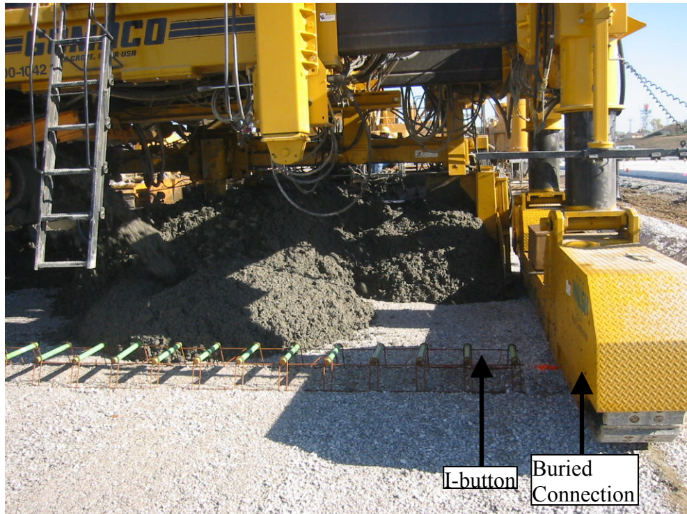
Figure 3.12: Covering of maturity sensor
