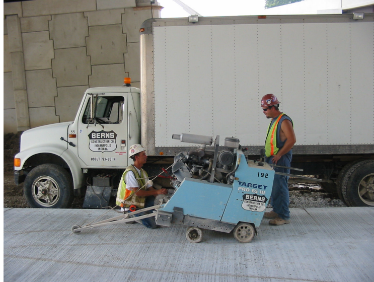
Figure 3.4: Conventional 65 horsepower wet-cut saw with 18 1/8" diamond blade
