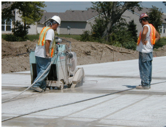
Figure 2.7: Conventional wet-cut saw
