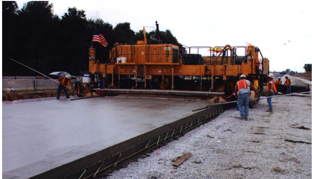
Figure 10-27 Finishing Pavement
