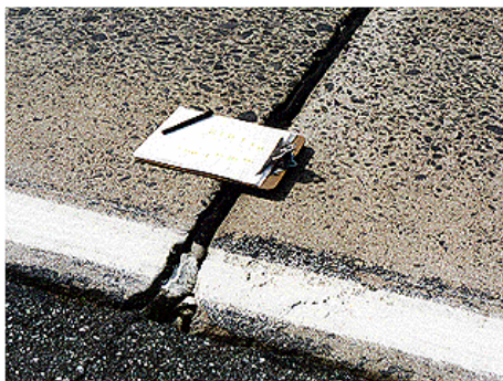
Figure 4-3 Faulting (Voigt 1996)
