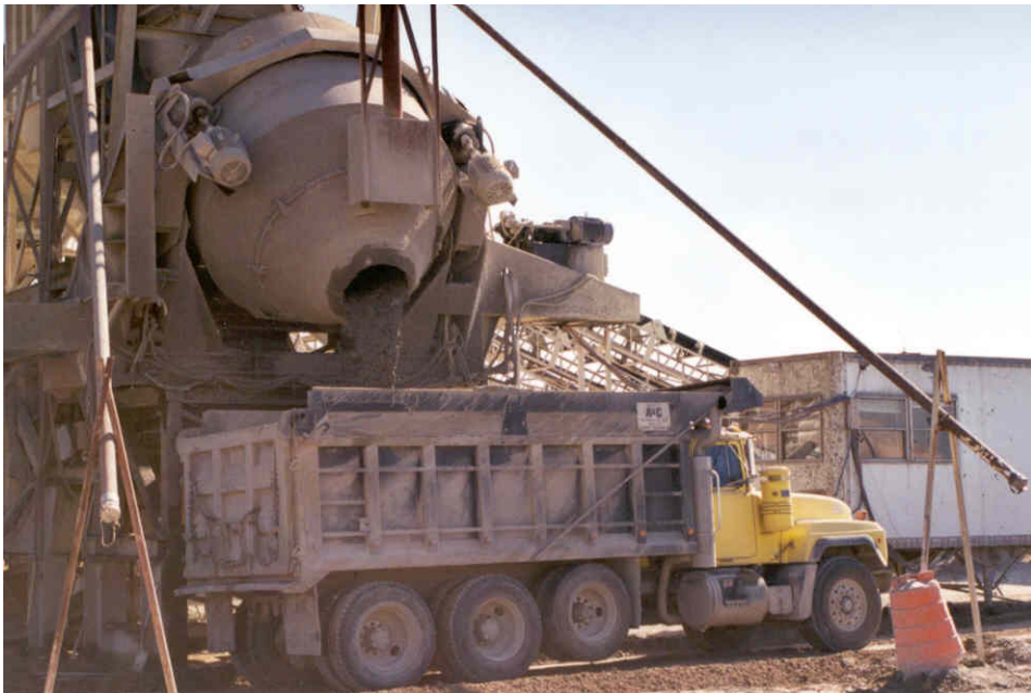
Figure 10-4 Fresh Concrete Ready for Transportation
