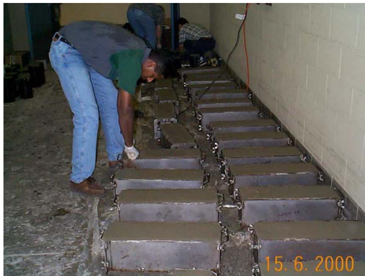
Figure 10-10 Finishing Beam Specimens
