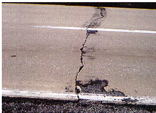
Figure 4-4 Transverse Cracking (Voigt 1996)
