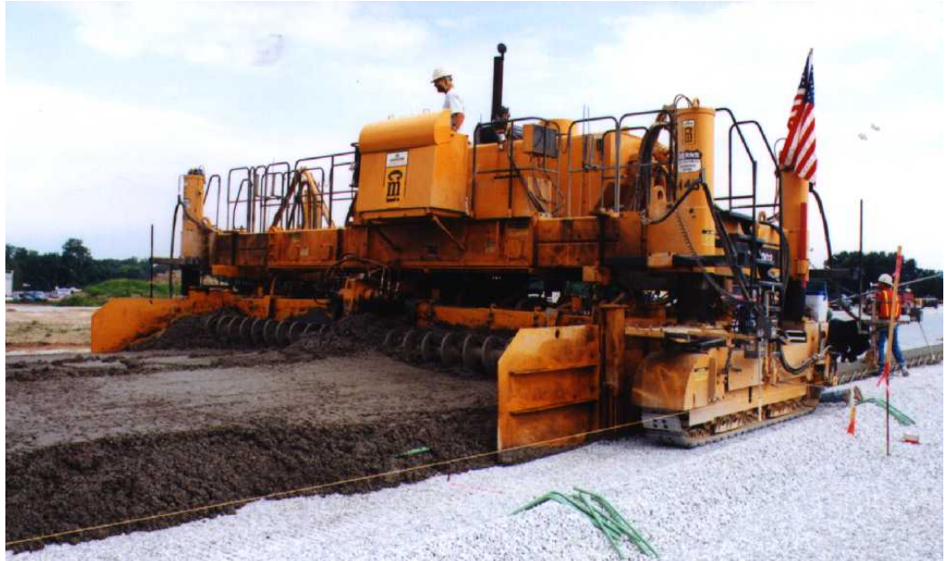
Figure 10-26 Vibrating Concrete
