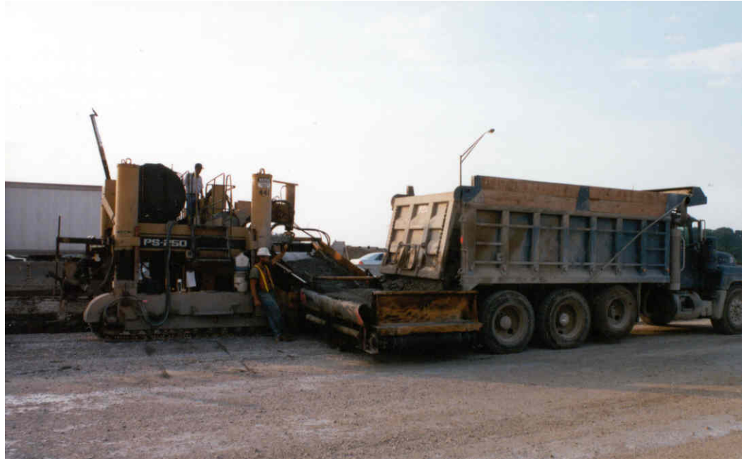
Figure 10-24 Concrete Dumped Onto Conveyor Belt
