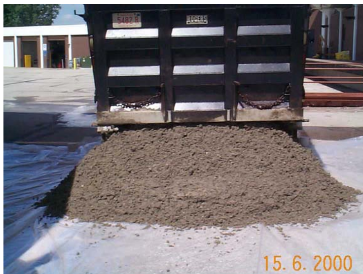
Figure 10-5 Fresh Concrete Delivered by Contractor
