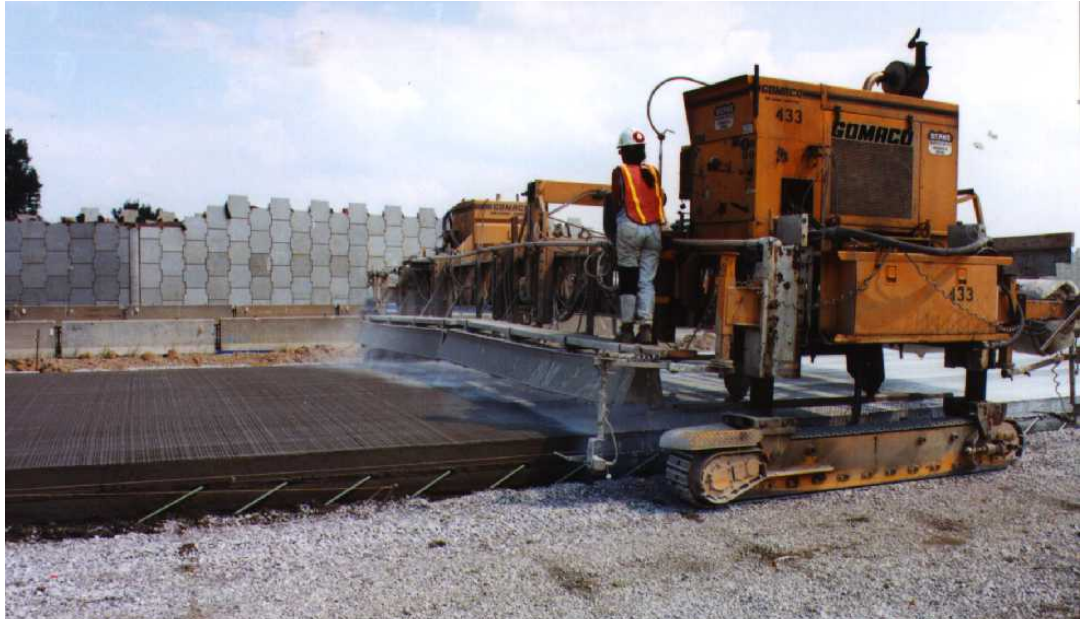
Figure 10-28 Tined Pavement is Covered with Curing Compound
