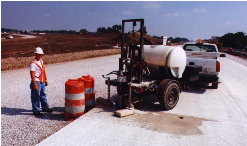
Figure 10-30 Obtaining Pavement Cores
