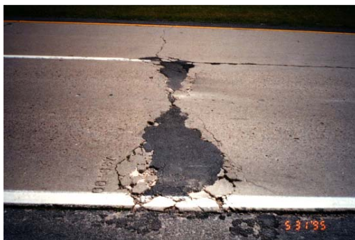
Figure 4-2 Spalling (Voigt 1996)
