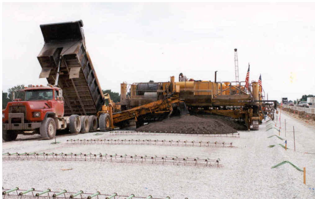
Figure 10-25 Concrete Spread Over Base
