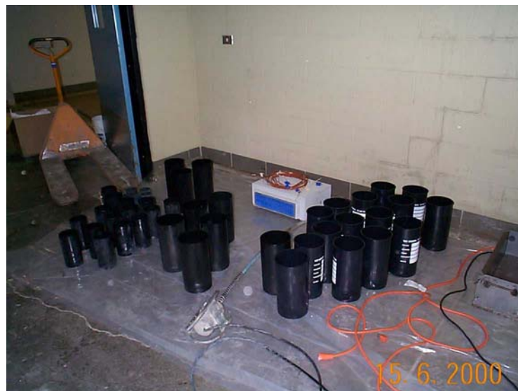
Figure 10-9 Cylinder and Beam Forms Inside Building
