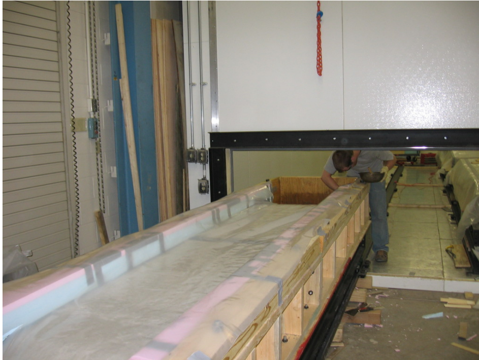
Figure 13-10 – Photo of Formwork Prepared for Large Scale Test Slab
