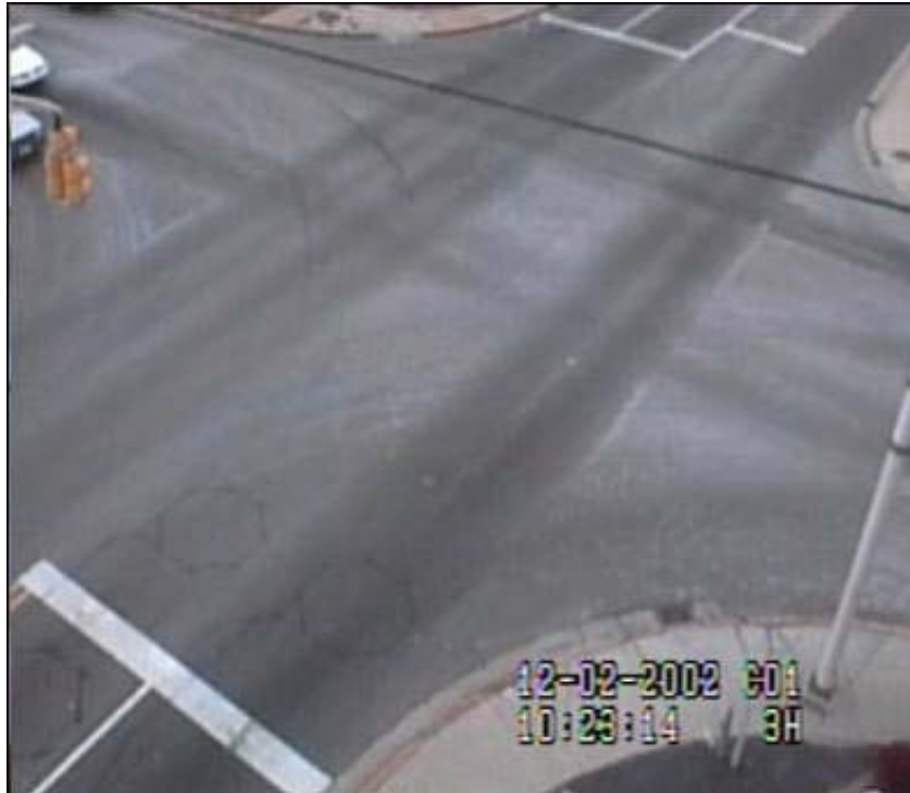
Figure 4-19: Field of View of SR-26 @ Earl Ave (No Shadow)
