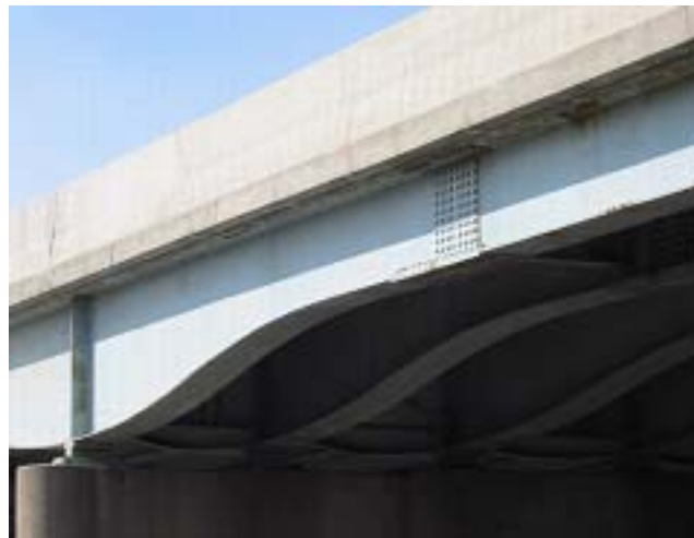
e) Bolted Splice Plate Connection
