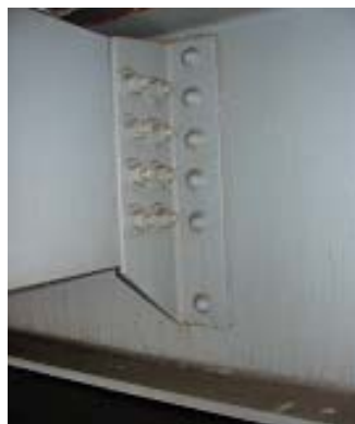
b) Riveted Diaphragm Connection
