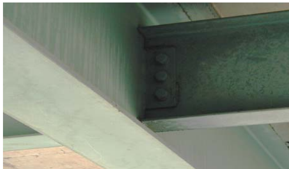
Figure 5.4 – Shear-Plate Connection at Diaphragm Section
