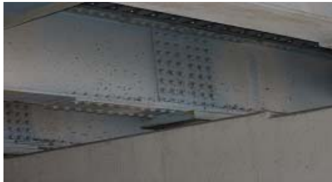
d) Bolted Splice Plate Connection
