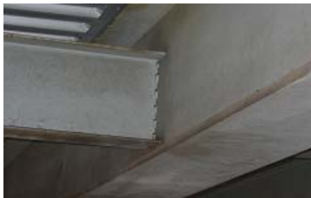
c) Intermittent Weld Diaphragm Connection
