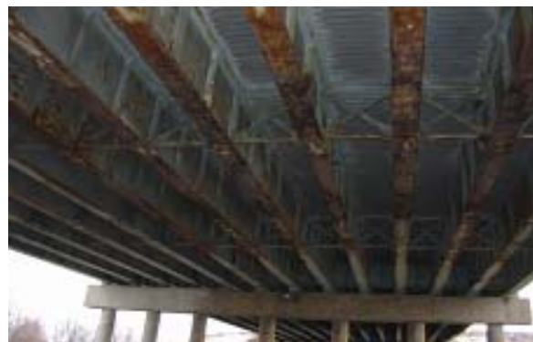
b) Diaphragm Framing
