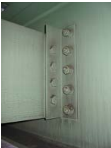
c) Bolted Diaphragm Connection
