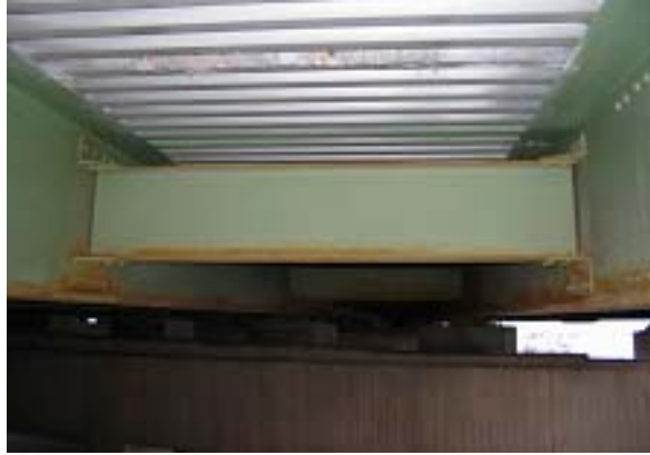
c) Riveted Diaphragm Connection
