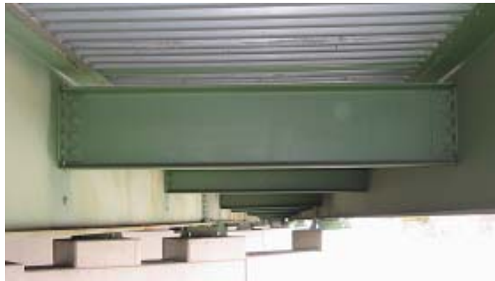
b) Bolted Diaphragm Connection
