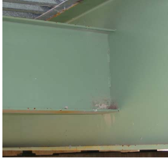
a) Intermittent Fillet Weld Diaphragm Connection
