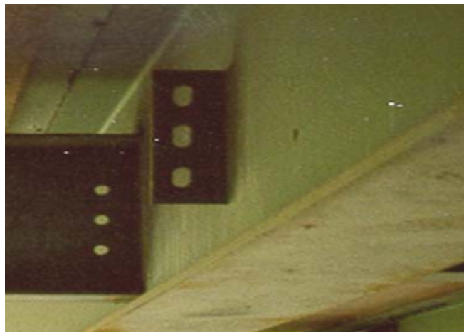
Figure 5.5 – Improperly Located Shear Plate
