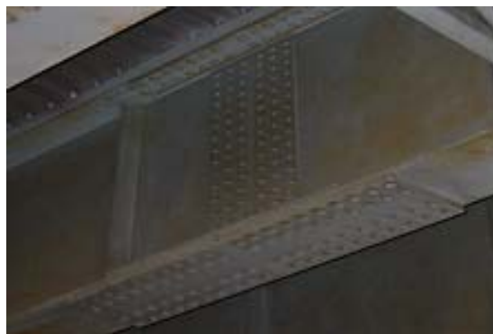
f) Bolted Splice Plate Connection
