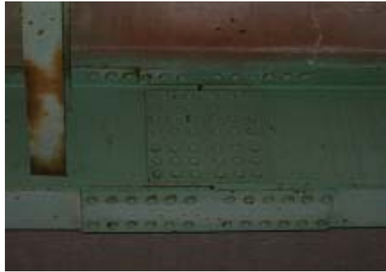
c) Bolted Splice Plate Connection
