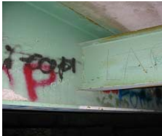
b) Intermittent Weld Diaphragm Connection
