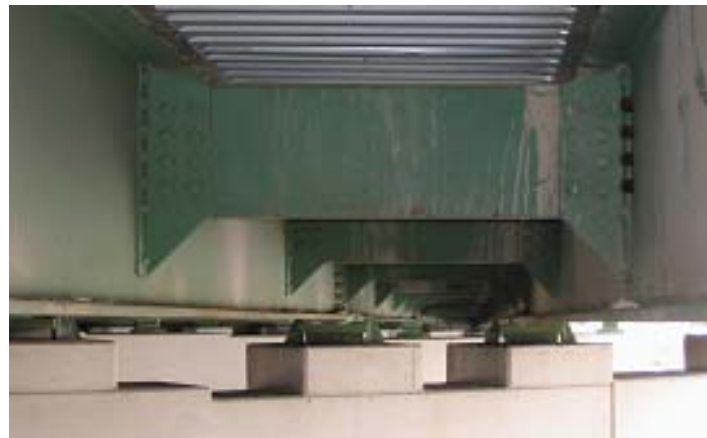
c) Riveted Diaphragm Connection
