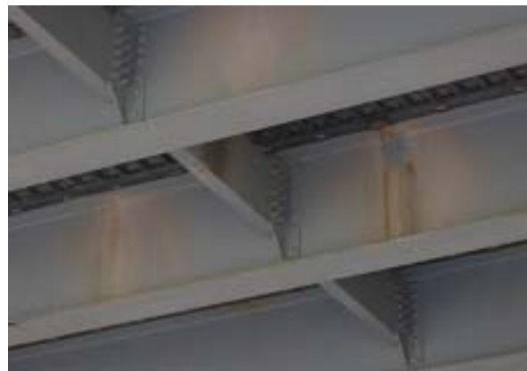
c) Riveted Diaphragm Connection
