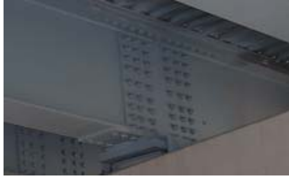
d) Bolted Splice Plate Connection
