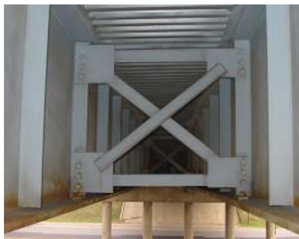
c) Cross-Frame Diaphragm
