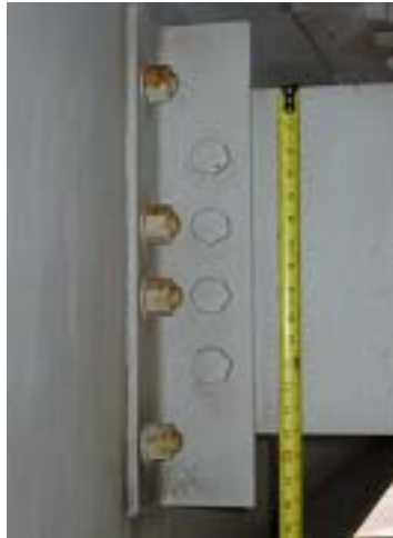
d) Bolted Diaphragm Connection
