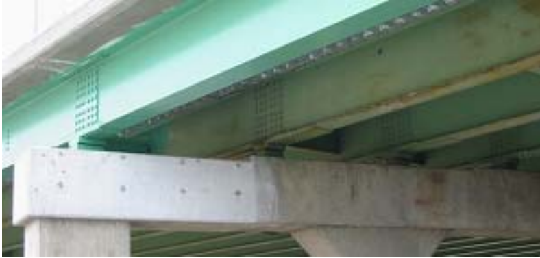
d) Bolted Splice Plate Connection
