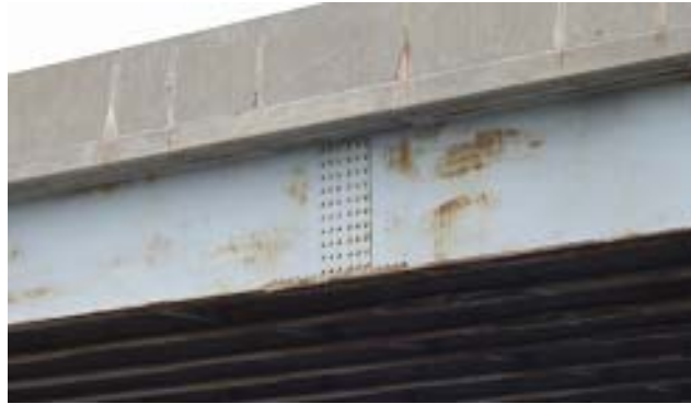
d) Bolted Splice Plate Connection
