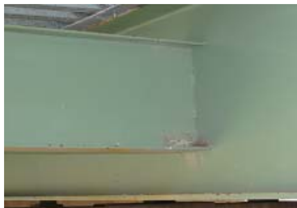
c) Intermitted Weld Diaphragm Connection
