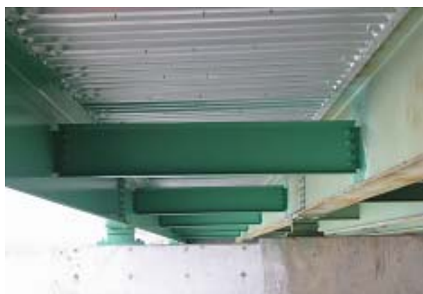
b) Bolted Diaphragm Connection
