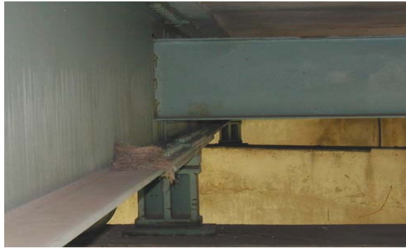
Figure 5.3 – Intermittent-Welded Diaphragm
