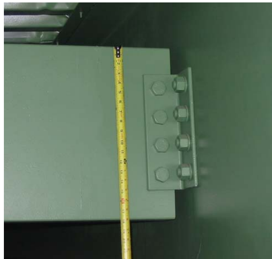
b) Bolted Diaphragm Connection
