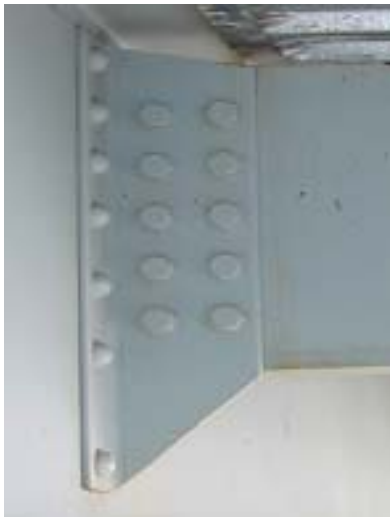
c) Riveted Diaphragm Connection
