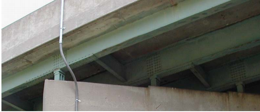
Figure 5.2 – Typical Bolted Splice Plate at Support
