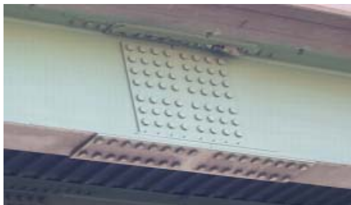
d) Bolted Splice Plate Connection
