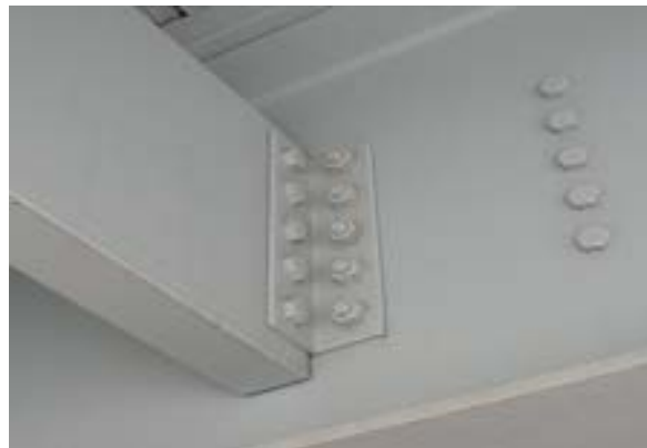
b) Bolted Diaphragm Connection
