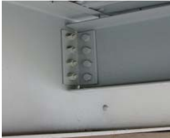
c) Bolted Diaphragm Connection
