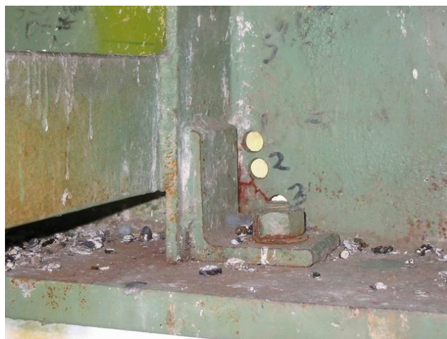
Figure 5.21 – Retrofit Angle Detail at Diaphragm Section
