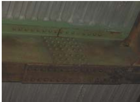
d) Riveted Splice Plate Connection
