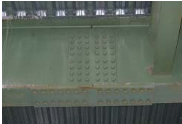
e) Bolted Splice Plate Connection
