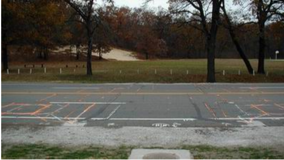
Figure 3.1 – WIM Sensors and Control Loops
