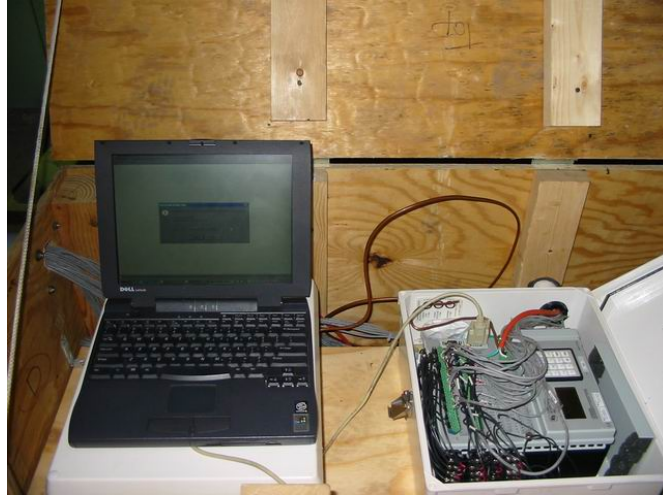
a) CR 5000 Data Acquisition System and Cable Wiring
