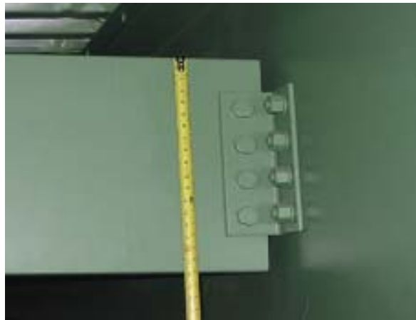
c) Bolted Diaphragm Connection
