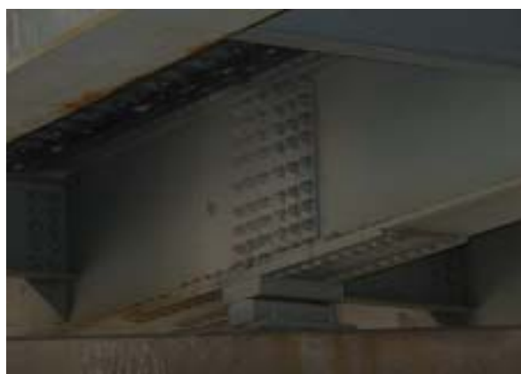
d) Bolted Splice Plate Connection
