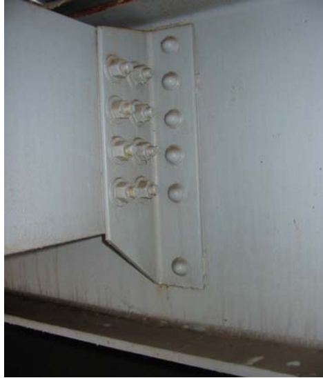
c) Riveted Diaphragm Connection
