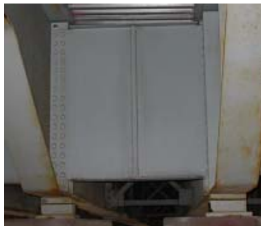
c) Jacking Frame at Middle Support
