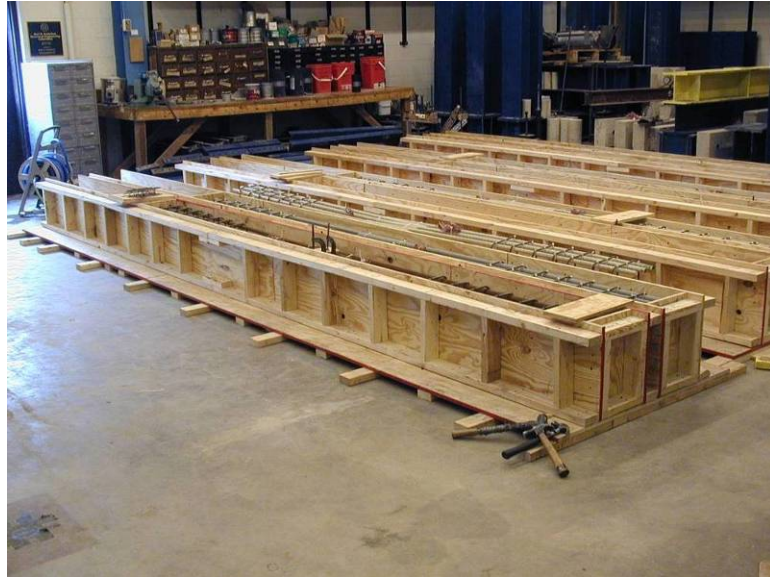
Figure 2.14 Assembled Formwork (Series I)
