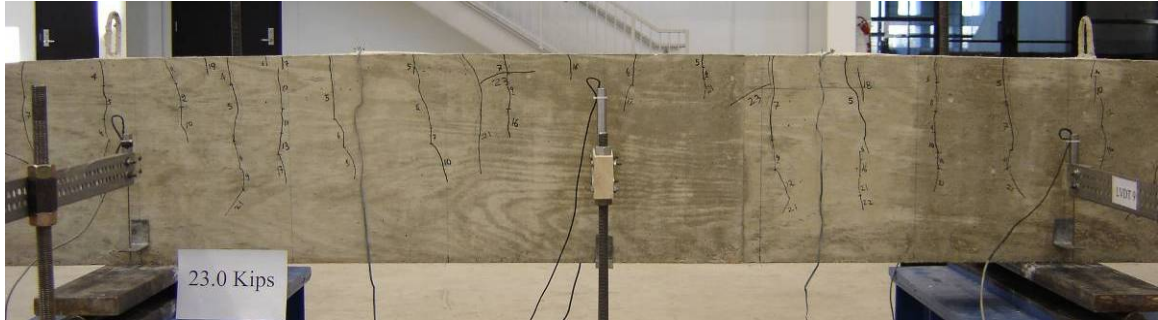
Figure 3.1 Cracking Pattern of Steel Reinforced Specimen Prior to Failure (Specimen B-S-5-24)
