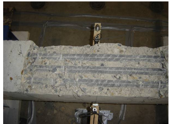
(b) Splice Region After Cover is Removed
