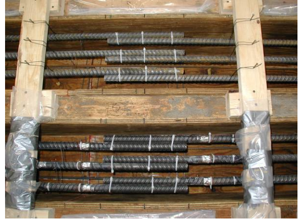
(b) Top Cast Bars in Splice Region
