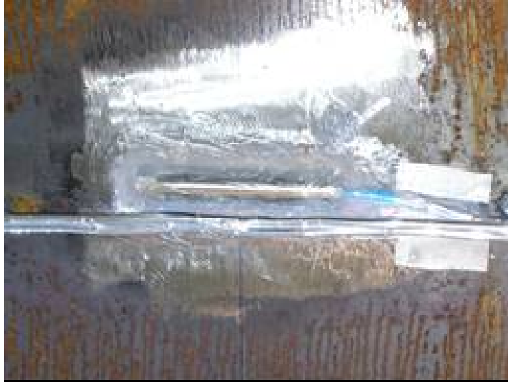
Figure A.3 Gage protected with steel cover and silicon caulking
