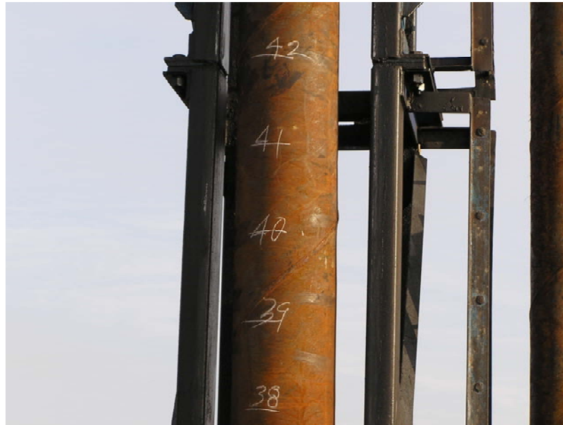
Figure A.5 Pile marked every 1ft for blow count records
