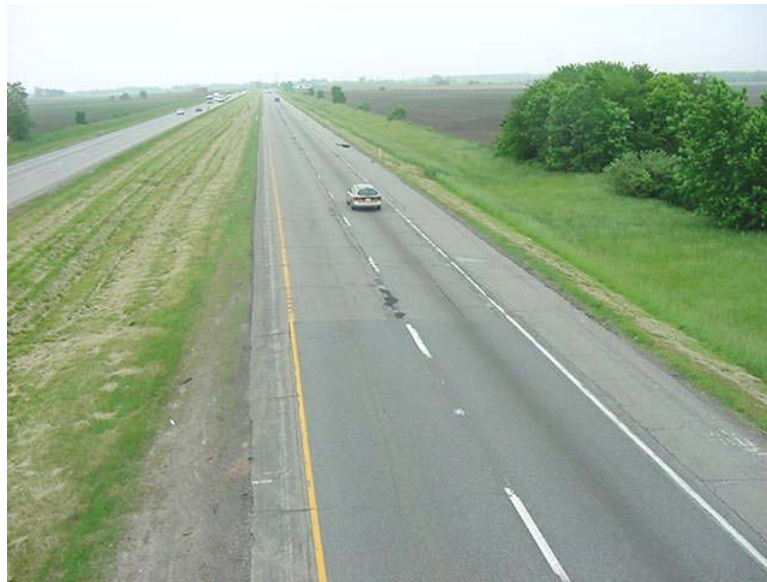
Figure 6-5 Interstate 65 Northbound at 113 th Avenue, Posted Speed Limit 65 mph
