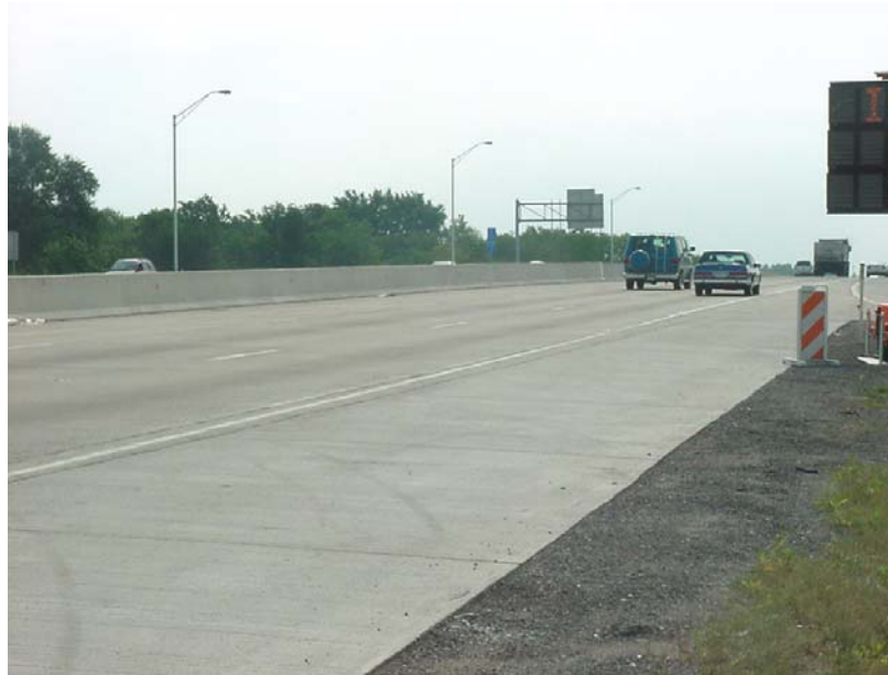
Figure 6-9 Interstate 65 Southbound at Ridge Road
