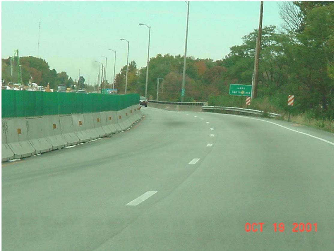
Figure 2-1 Roadway conditions of I-55 during reconstruction of Lake Springfield Bridges(10/19/01)
