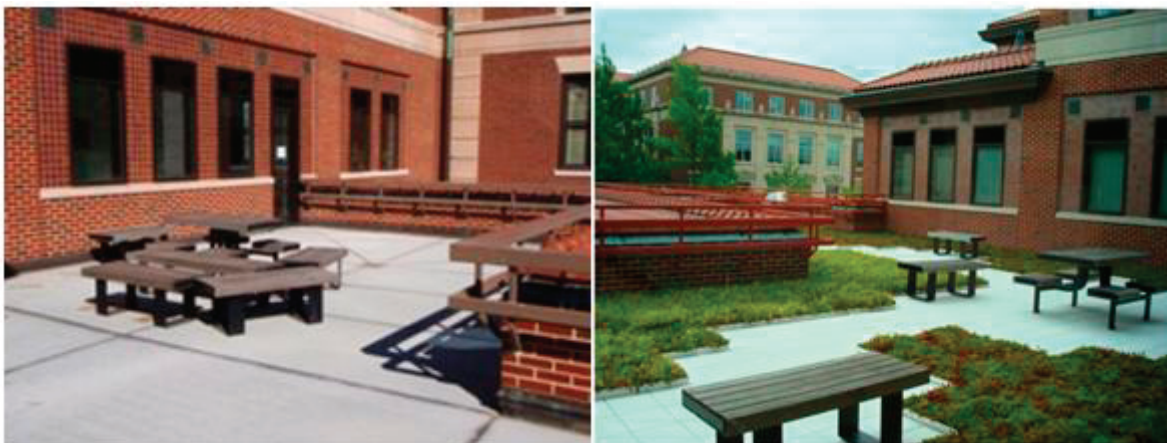
Figure 1: Schleman Hall before and after green roof installation
