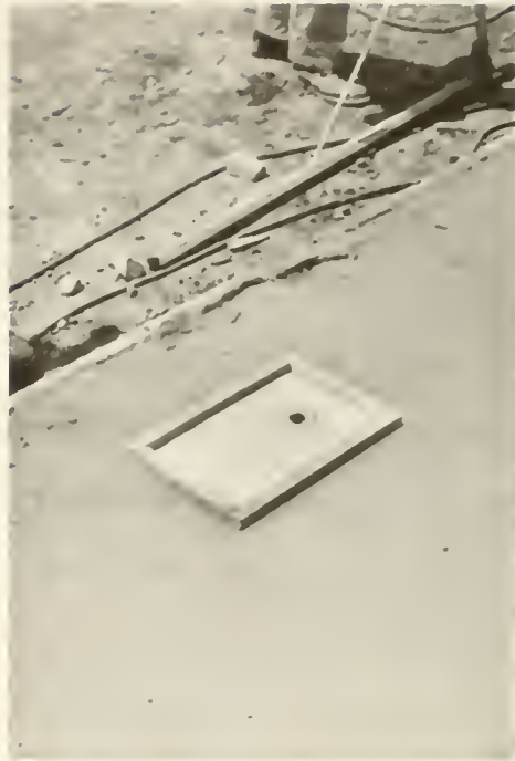
Fig. 4. Sheet Metal Tray Positioned Over Hole.
