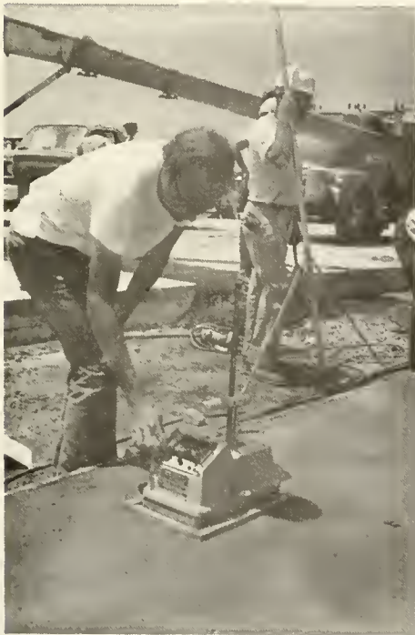
Fig. 5. Meter in Place With Probe Extended Into Hole. Test Underway.
