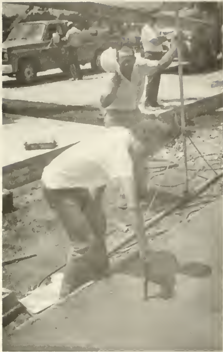
Fig. 3. Forcing Rod Into Fresh Concrete to Form Holes.
