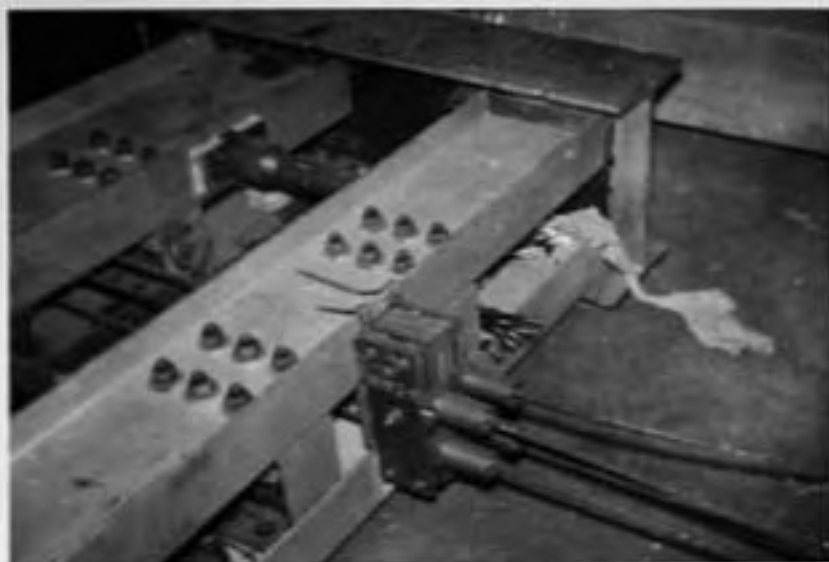
FIG. 7 JACKING END OF PRESTRESSING BED
