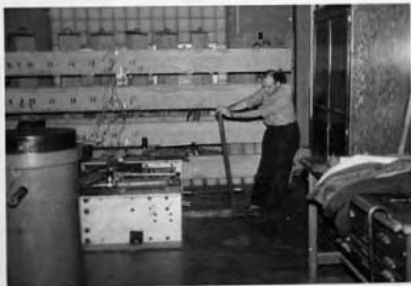
FIG. 8 PRELIMINARY STRESSING OF STRANDS
