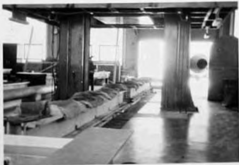
FIG. 13 AFTER POURING, BEAMS COVERED UP
