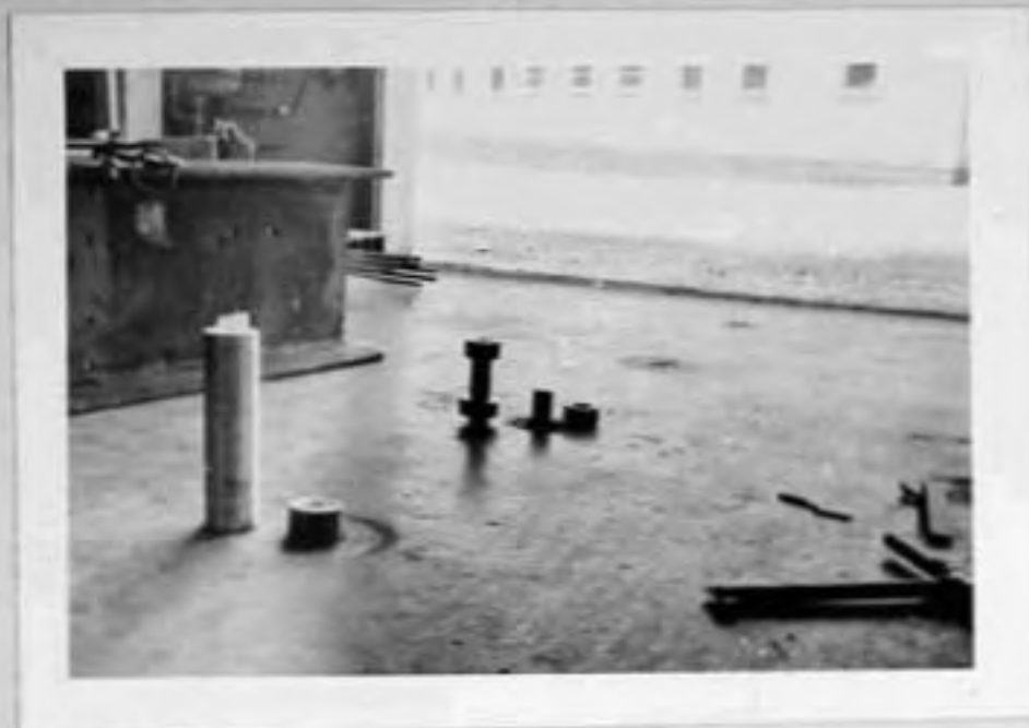
FIG. 3 PLUG AND TIEDOWN BOLT FOR PRESTRESSING BED
