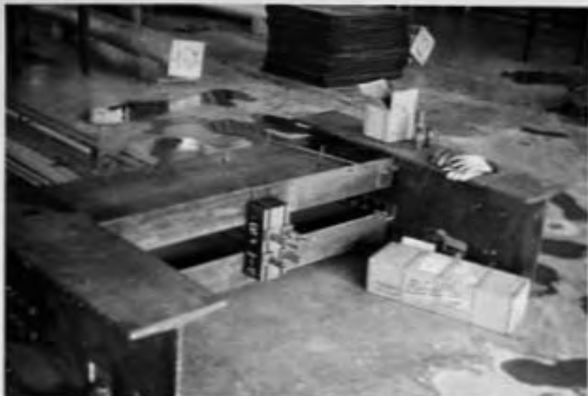
FIG. 5 FIXED END OF PRESTRESSING BED
