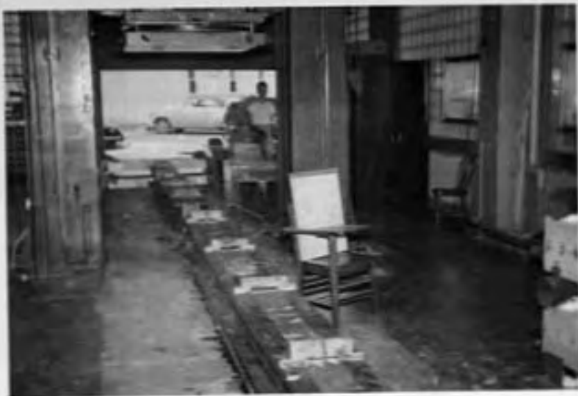
FIG. 12 BEAMS IMMEDIATELY AFTER POURING
