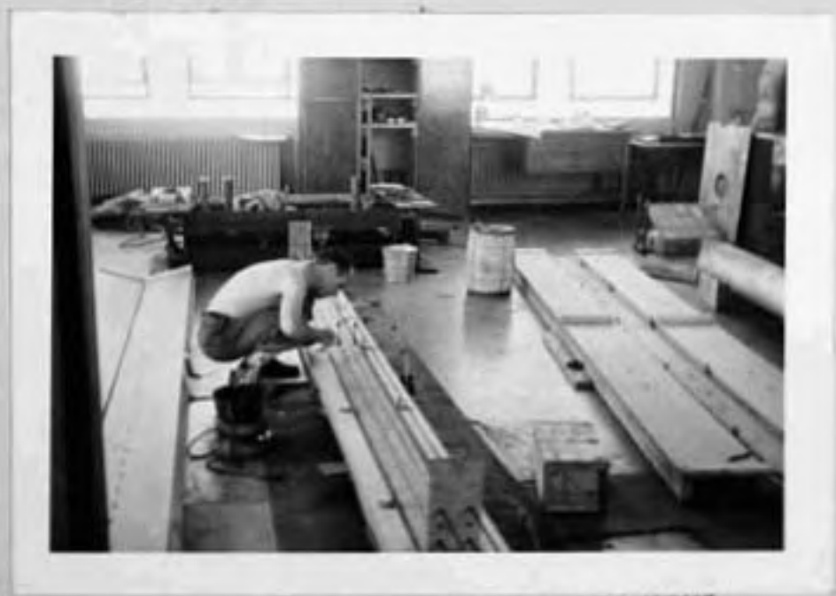
FIG. 17 BEFORE ASSEMBLING OF FORMS
