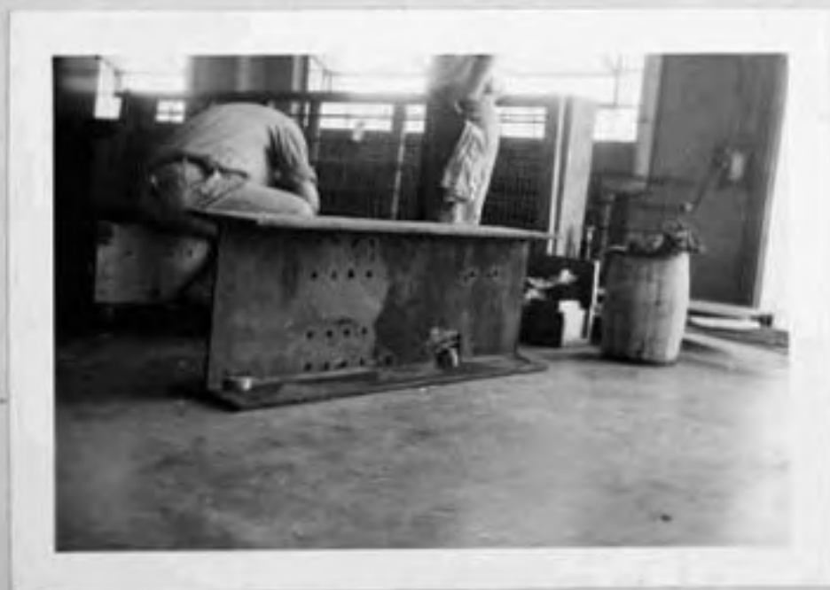
FIG. 4 GIRDER FOR PRESTRESSING BED
