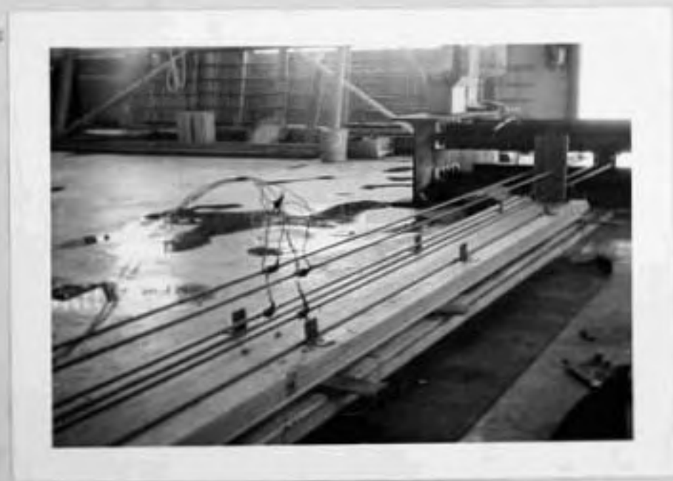
FIG. 11 SHIMMING OF BOTTOM SECTION OF FORM
