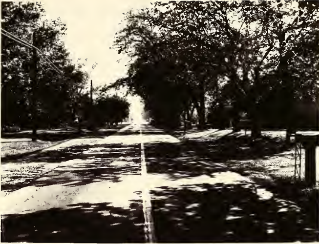
SITE E— 21 ST. STREET, INDIANAPOLIS
