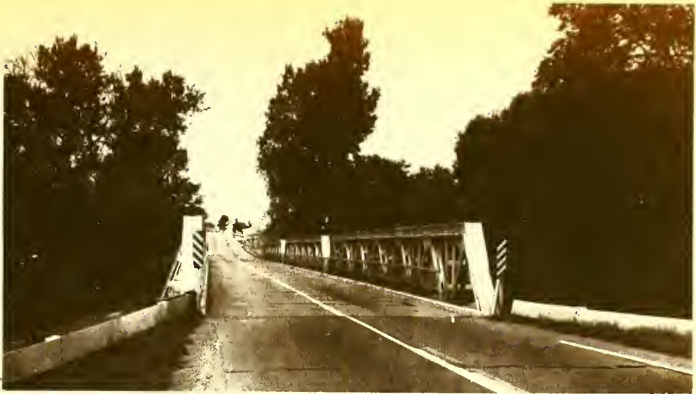
Entrance to bridge from south.
