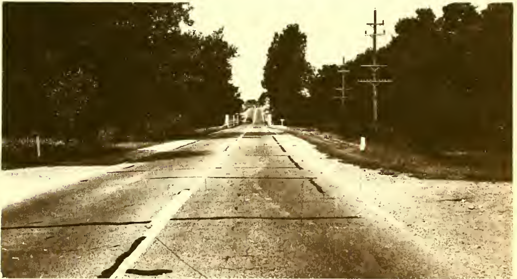
Approach to bridge from south.
