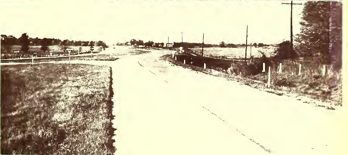
Top: Center of intersection, looking north. S.R. 431 in right background. Center: Merging area, looking north on U.S. 31. Bottom: Approach to merging area from S.R. 431.
