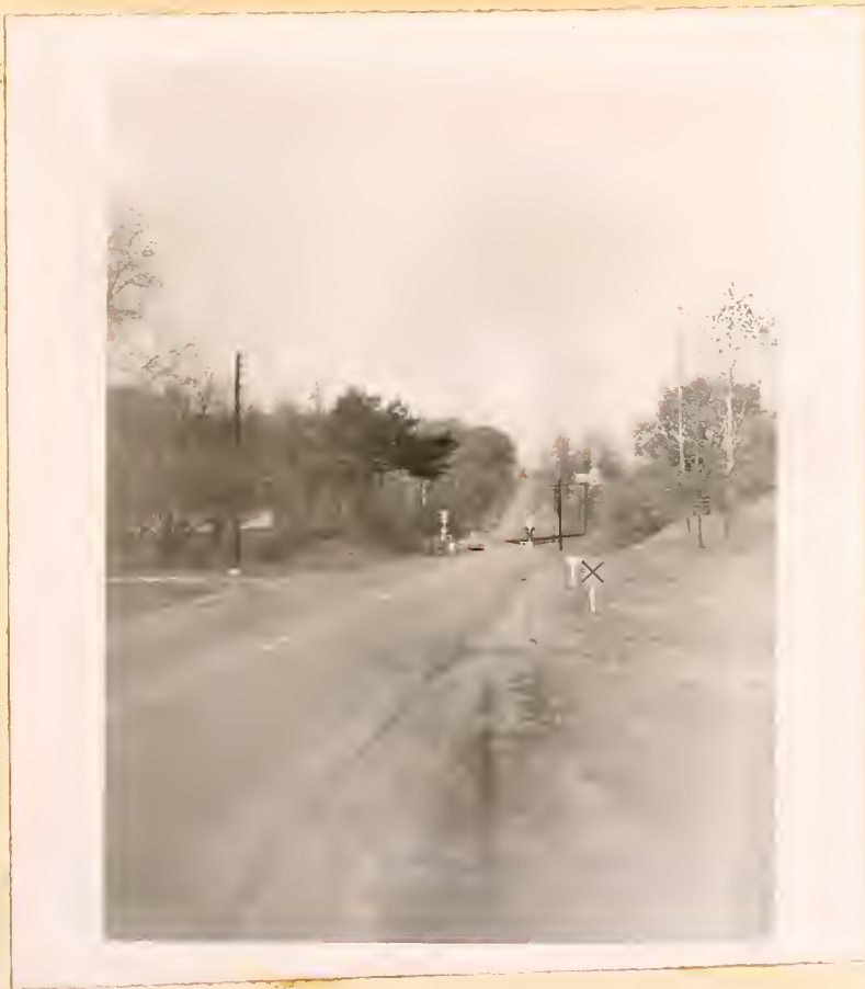
Inadequate sight distance and alignment typical of earlier construction practices restrict free and safe movement of vehicles.
