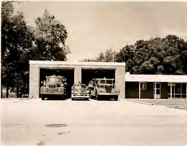
Highways are indispensable during local emergencies for the movement of police and fire fighting equipment.
