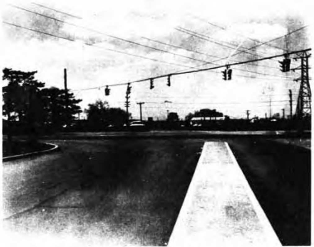
FIGURE 14 TEAL ROAD - POOR APPROACH ALIGNMENT
