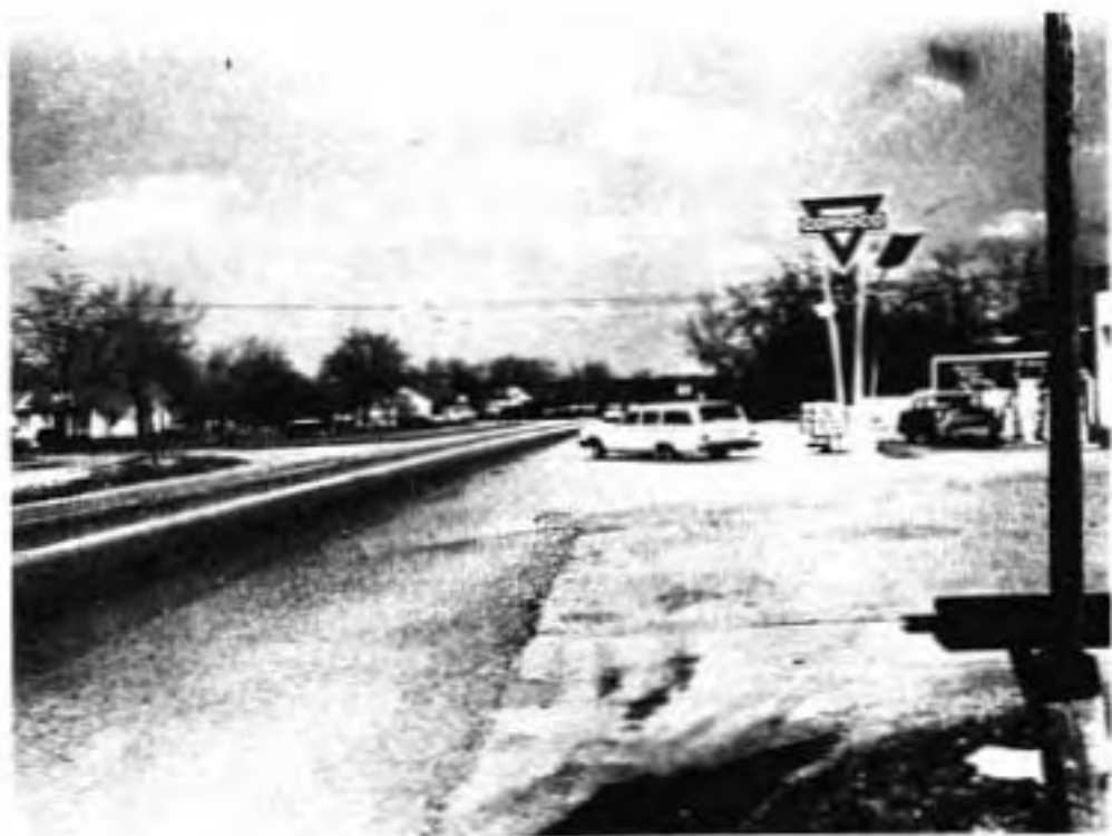
FIGURE 22 NORTHEAST QUADRANT OF INDIANA 25 INTERSECTION - POOR DRIVEWAY DELIMITATION
