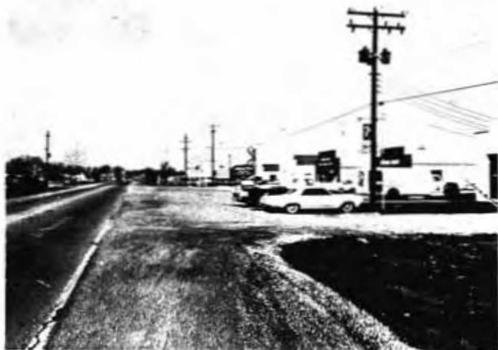
FIGURE 29 EXAMPLE OF POOR DRIVEWAY DELIMITATION
