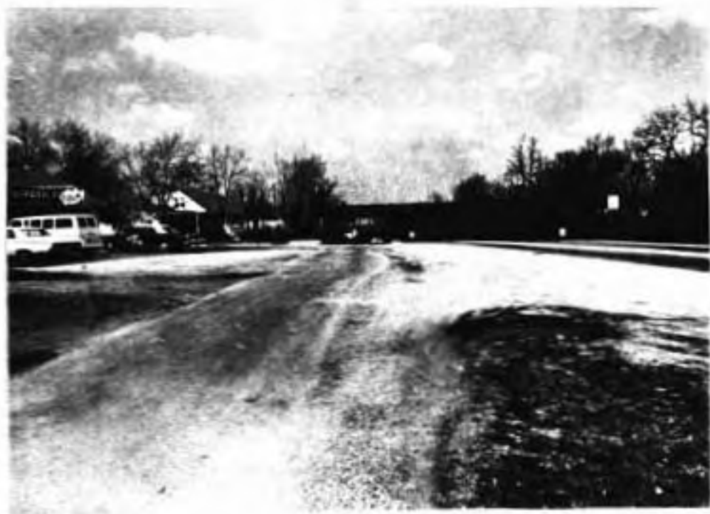
FIGURE 21 NORTHWEST QUADRANT OF INDIANA 25 INTERSECTION - POOR DRIVEWAY DELIMITATION
