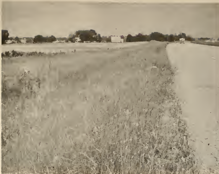
Fig. 7. Portion of the I-74 photographed in the 3rd week of June, 1974. Grass is 18 to 24 inches high and at the proper stage for the first mowing.
