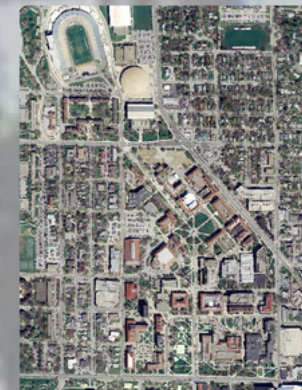
"WPA Temporary Building" removed to make way for new Bell Armstrong Engineering Building, next to Civil Engineering. Stadium Mall returns to single lane, emergency traffic only. Can you find the old smoke stack shadow? (It's gone.) However, there is a shadow cast by the newly constructed Bell Tower. Can you find that? Fred and Mary Ford Food Court is added west of Cary Quad. Note the newly renovated Football Stadium. Color makes the Math Building shadow more distinct. The old fountain, formerly in front of Howde Hall of Administration, finds a new home between Matthews Hall and Stone Hall.
