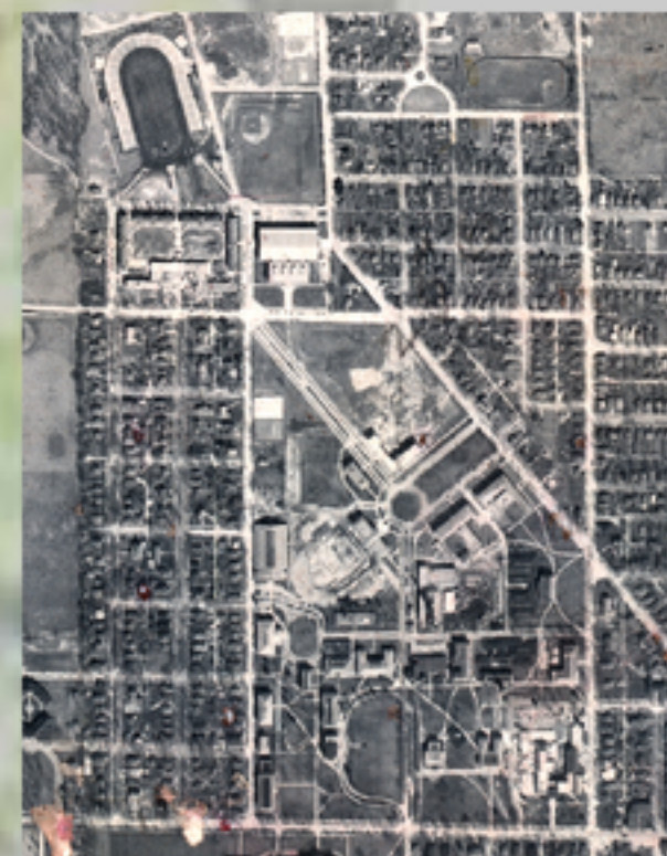
Stadium Mall becomes two lanes. Howde Administration Building appears in this aerial photo as well as Chemical and Metallurgical Building across from Pharmacy. Cary Quad and Field House appear under construction. Cary Quad and Field House show up in this photo. Can you find the old smoke stack shadow?
