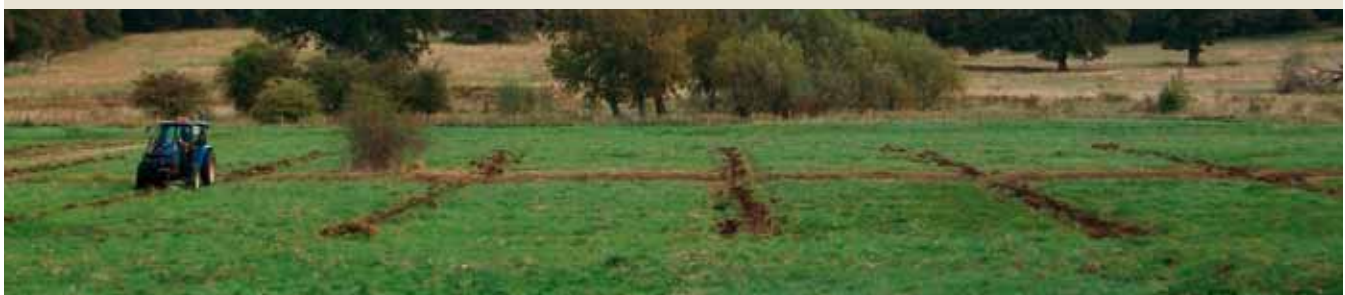
A network of shallow cross drains created to facilitate removal of water from the top layers of the soil to preventing soil waterlogging and anoxia. © RNRP
