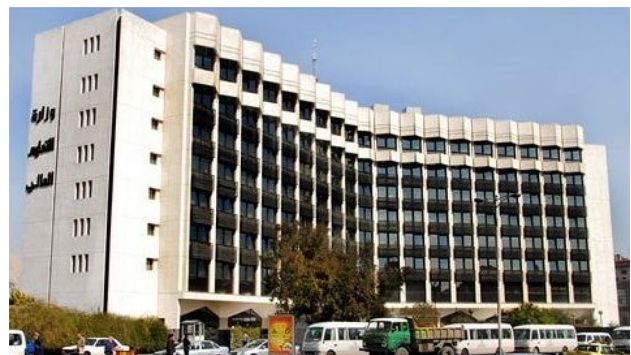
Fig. 1 Building of the Ministry of Higher Education (MHE) in Syria
